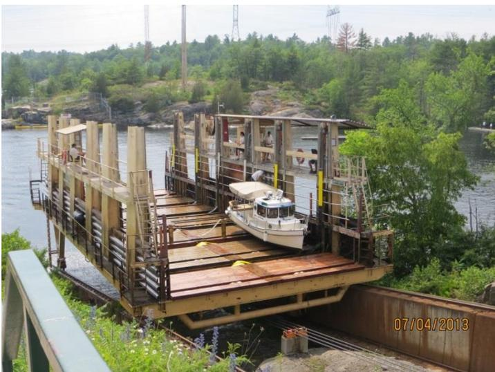
Figure 2.5: Marine railway ([mvislandhopper.blogspot.nl](http://mvislandhopper.blogspot.nl))
