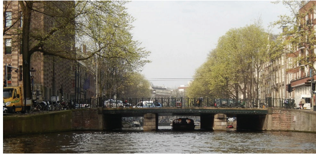
Fig. 1. Bridge on wooden pile foundation in Amsterdam/Netherlands
