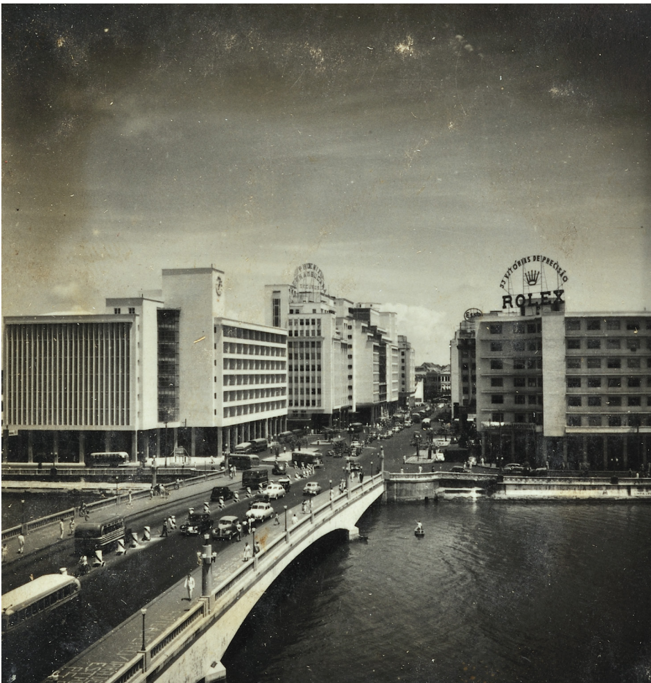
Guararapes Avenue with the arcades on the ground floor and progressive setback on the higher levels, artifices originated from the 1919 law that allowed higher buildings in the centre.
