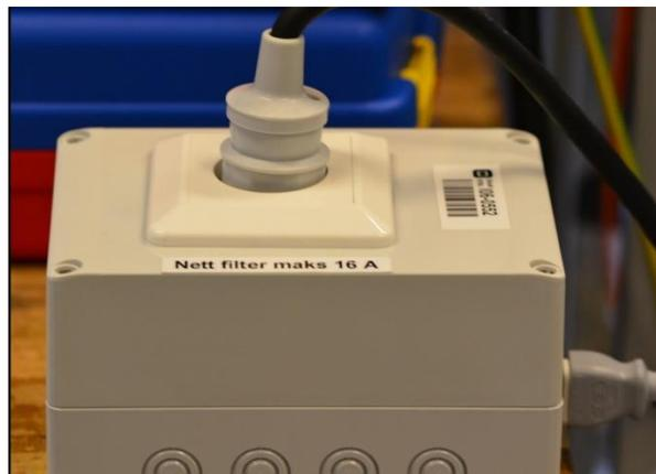
Figure 30. Grid side filter used with a maximum current flowing of 16A.
