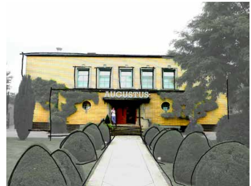
Fig. 85 Main entrance with non-functional greenery [from: Nienoord, 2013]
