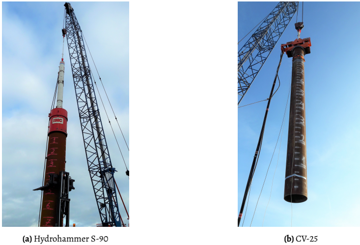
Figure 1.2: (a) Impact hammer and (b) axial vibratory device mounted on the top of tubular piles from the GDP field campaign.
