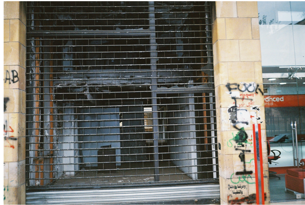
Figure 23: A building near the city centre. Buildings tent to be more damaged the further away from the facade, due to pressure building up inside the buildings after the shock-wave, exploding them from the inside out. Personal photograph from case study.
