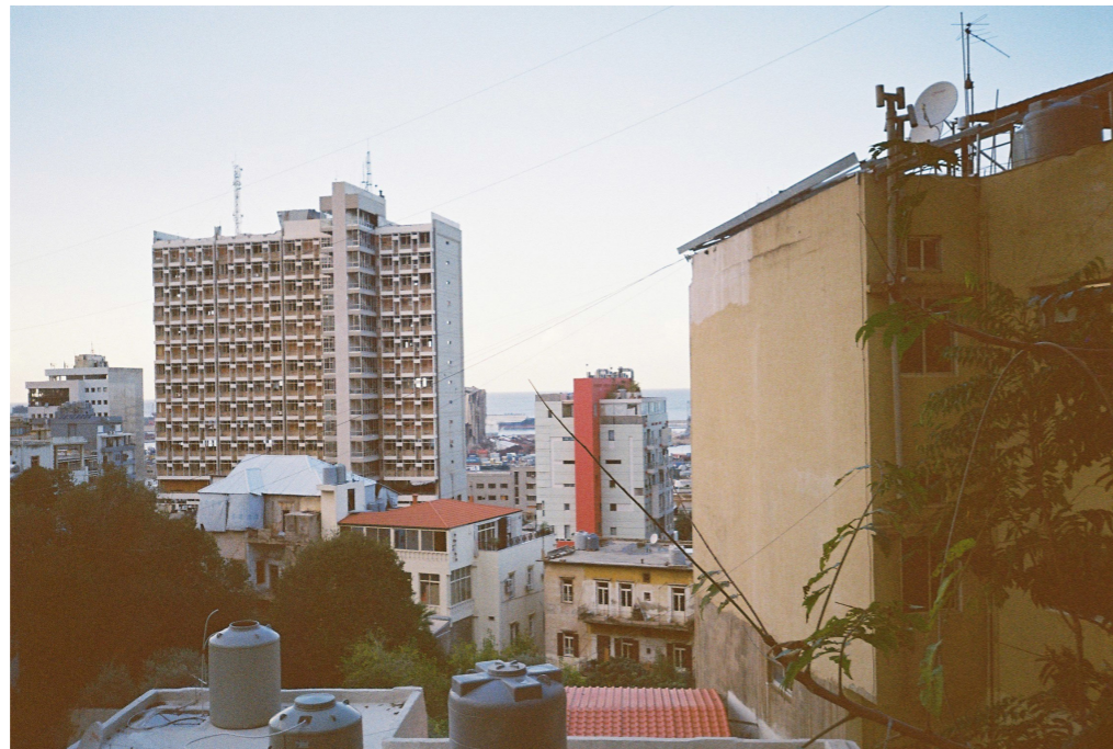
Figure 30: Right behind the electricity building on the left, the destroyed silo, which was standing right next to the explosion site, can be seen. Personal photograph from case study.
