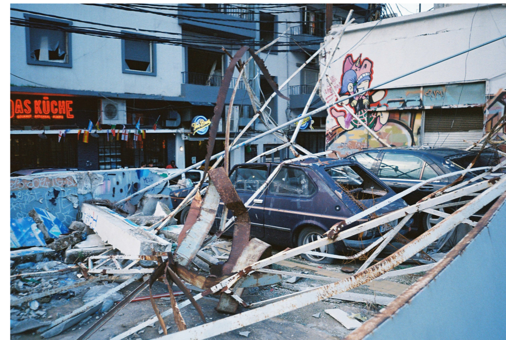
Figure 26: Cars crushed by steel, behind the gas station, as shown in the previous photograph. After 2,5 years these have not yet been removed. Personal photograph from case study.
