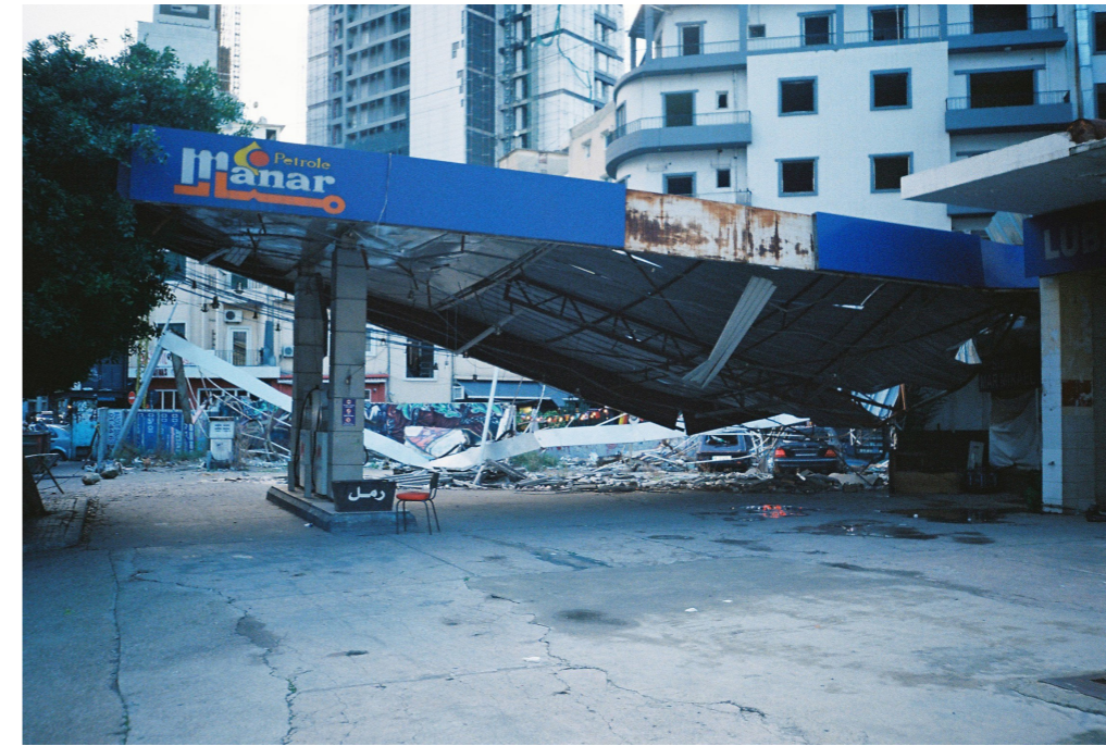
Figure 25: A destroyed gas station on Armenia Street. Close to the plot of this research. Personal photograph from case study.
