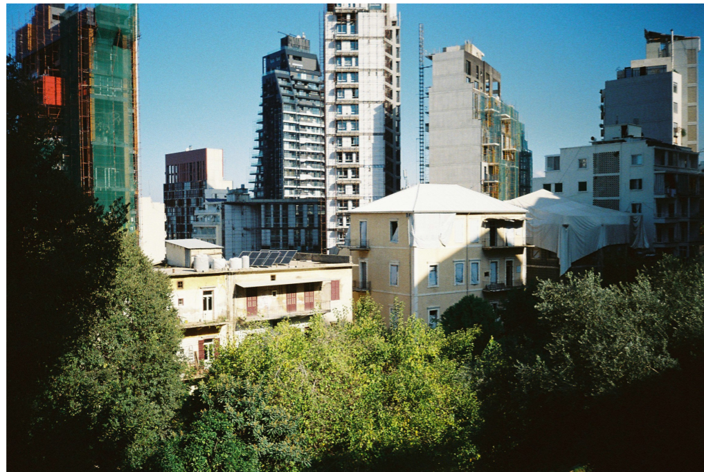
Figure 34: Heritage buildings right across from the plot of this research, covered with sheets to avoid further damage by rainfall. Personal photograph from case study.
