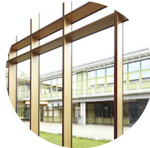
Timber curtain wall
