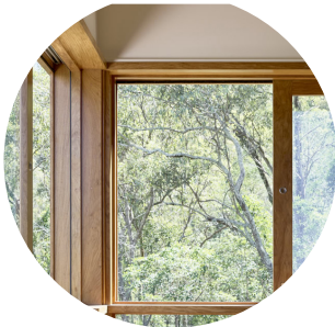
Timber window frame
