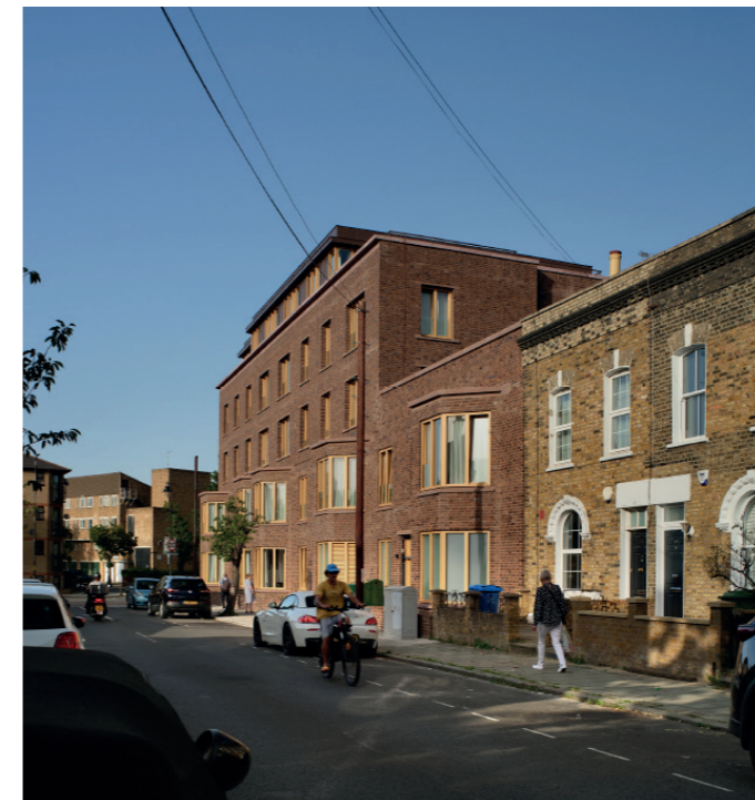
Facade follows street pattern
