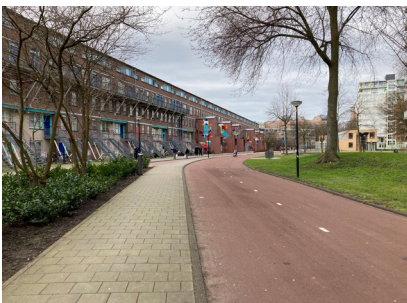
Footpath, bicycle-path & highway North-east ≈ 1970
