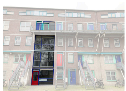
Glass facade North-east facade 1984
