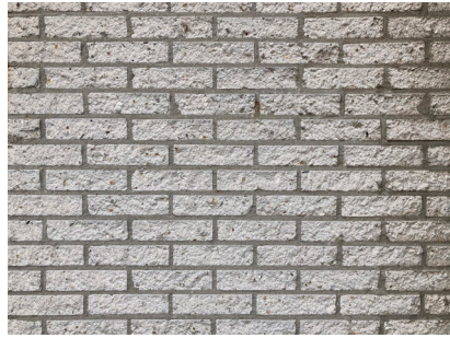
White brick Cladding Facade, North-east 1982
