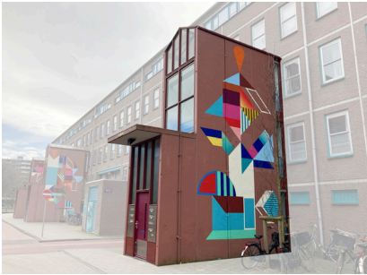
Stairwell entrance North-east facade 1984
