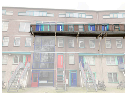
Balcony North-east facade 1984
