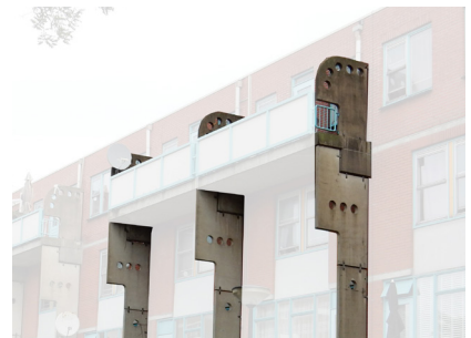
Concrete slabs South-west facade 1982
