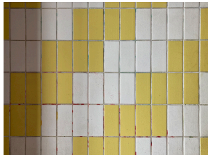
Yellow & white tiles Cladding Underpasses 1982 - present day
