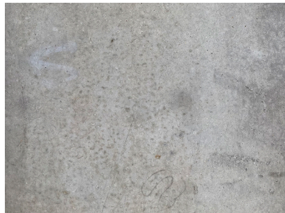
Semi smooth concrete Components Balconies & concrete slabs 1982 - present day
