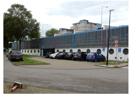
Parking garage South-west 1982
