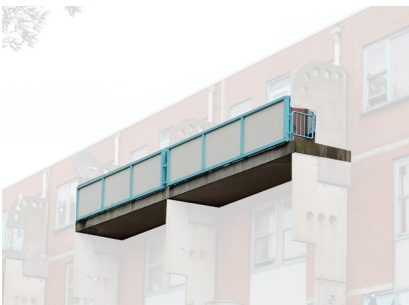
Rectangular balcony South-west facade 1982
