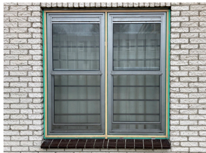
Double glazed windows Window frame Window 1982 - present day
