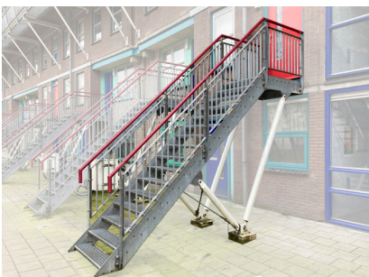
Exterior staircase North-east facade 1984
