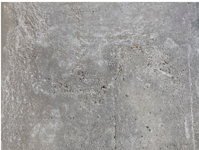
Raw concrete Structure Full building 1982 - present day
