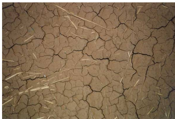
Figure 1.1: Detail of a house in New Mexico, USA [Schlangen].
