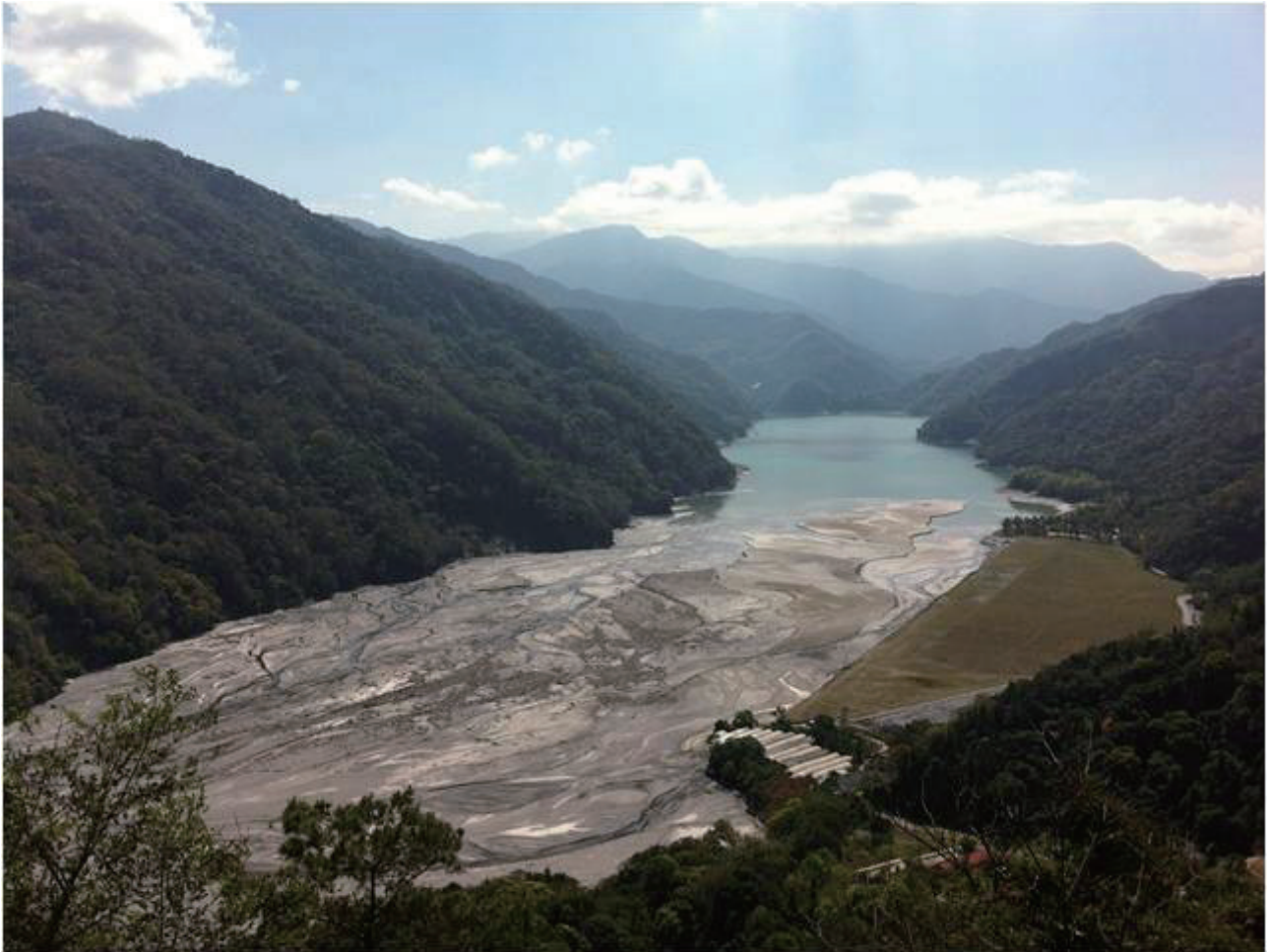
fig.09 Wushe ( 霧社 ) Reservoir, now 65% filled with sediment. Source: Taiwan Academy of Ecology epaper (2013) [Online] http://enews.url.com.tw/ [accessed 20. Feb. 2017]
