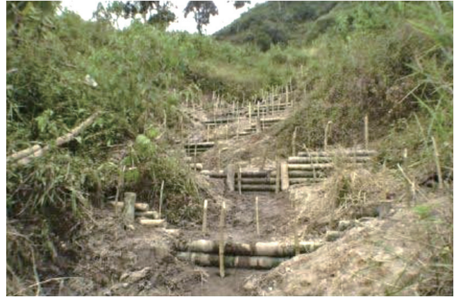
fig.71 Simple construction stabilize the slope. Source: Report of "Rehabilitar la Montana", municipality of Medellin.
