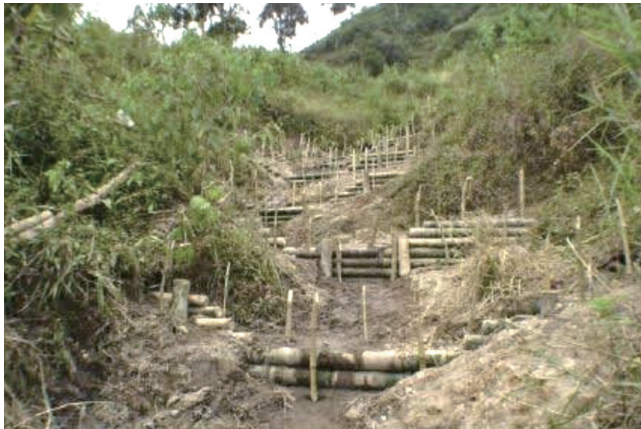
fig.126 Photo and diagram of slope stabilization structures. Source: Report of "Rehabilitar la Montaña", municipality of Medellín.
