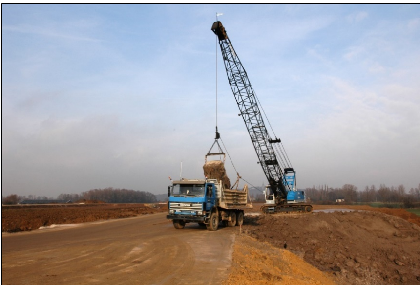
Figure 10. Storage yard (in Dutch 'kleidepôt') where extracted clay is stored, often closely located to the ceramic plant. Source: (KNB, 2020).
