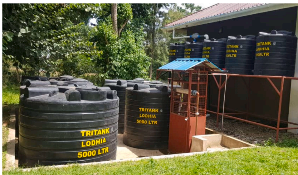
Fig. 4. Pilot demonstration of RWH in Arusha. (Source: Author).
