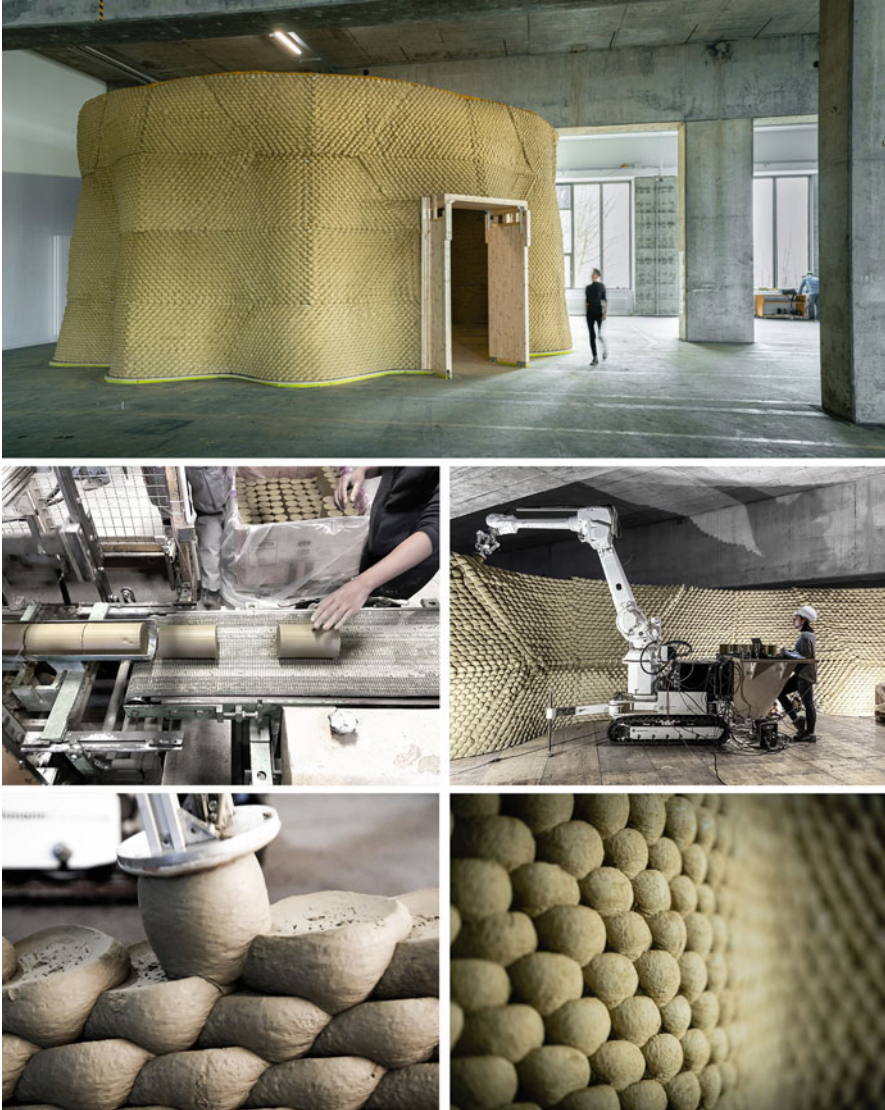
Fig. 9.3 (i) The Clay Rotunda is a cylindrical structure constituting the outer, soundproof shell of the electroacoustic auditorium SE MusicLab. (ii) The soft bricks were produced externally with an industry partner. (iii) The robotic pressing process was realised with the IF, which could be relocated on a temporary scaffold to realise a two-story structure. (iv) Detail of structure showing the bonding and interlocking between adjacent elements. (© Gramazio Kohler Research)
