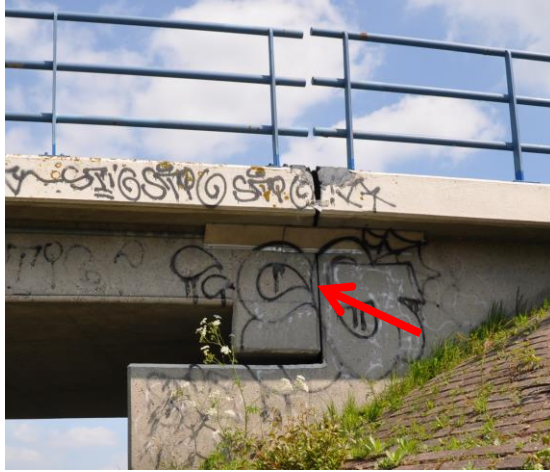
Fig. 11 Expansion joint at the South side of viaduct Zijlweg.
