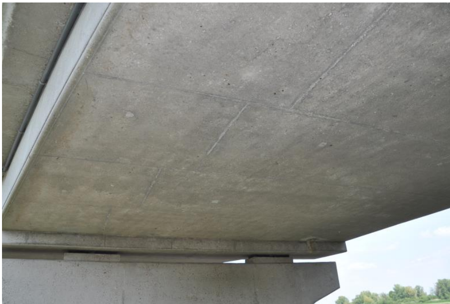
Fig. 9 Bottom of deck.
