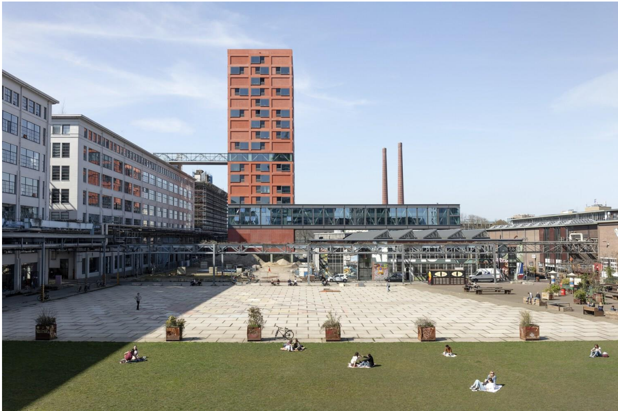
Figure 6.4: The tower of Haasje Over and its two bridges, one connecting it to the building beside it (left) and the other consisting of 48 maisonettes spanning over the old industrial hall (right). (Source: van der Burg, 2021)
