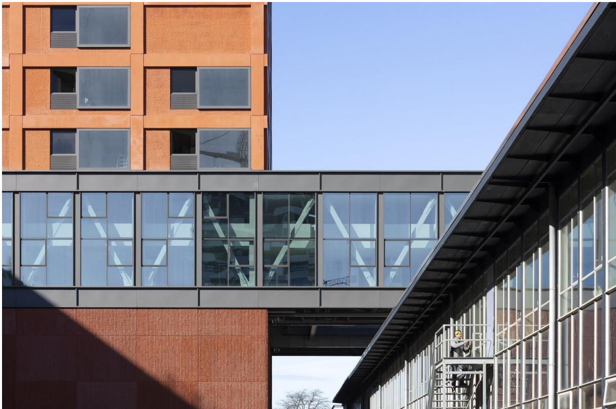
Figure 6.5: The maisonettes in the steel bridge construction of Haasje Over. (Source: van der Burg, 2021)
