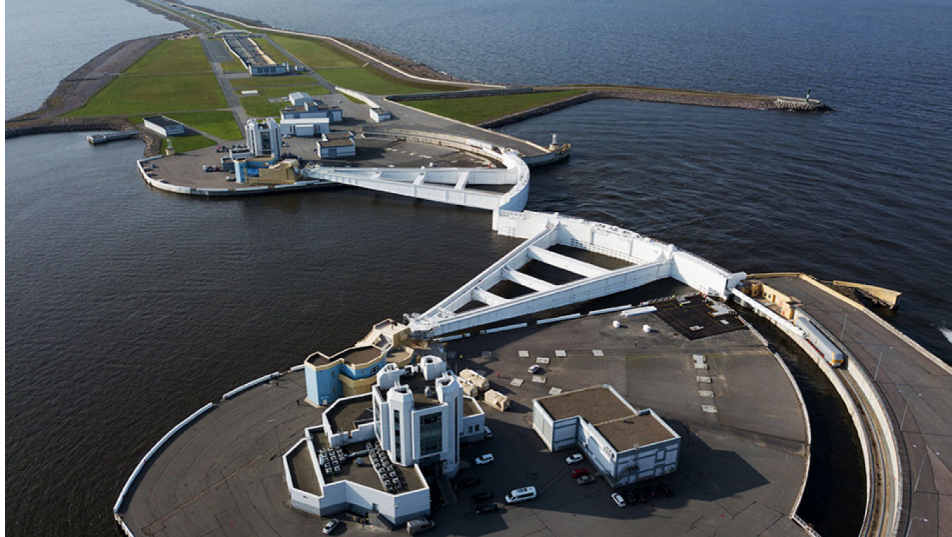
Figure 2.2: The S-1 navigation pass, St Petersburg Flood Protection Barrier (Kozin, 2024)
