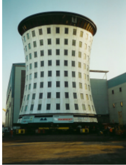
Figure 2.16: 'De Bolder' transported as a whole over to its final location.
