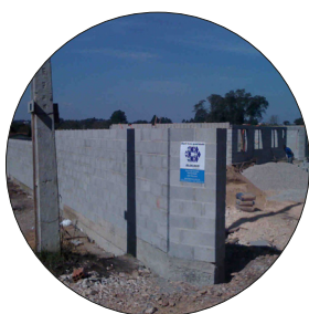
structural walls: blocos verdes
