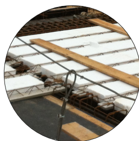
floors: recycled concrete + EPS
