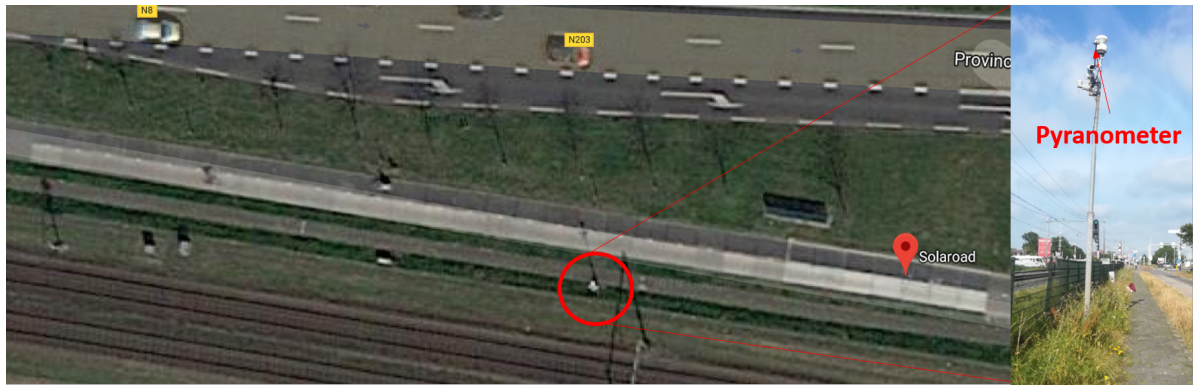
Figure 3.20: Location of the pyranometer mounted on the TNO SolaRoad in Krommenie
