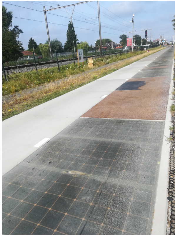
Figure 2.5: TNO SolaRoad pilot site in Krommenie (July 2019)
