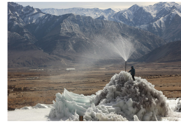
Pipeline connects the ice stupa to a source on higher ground, drawing water downhill
