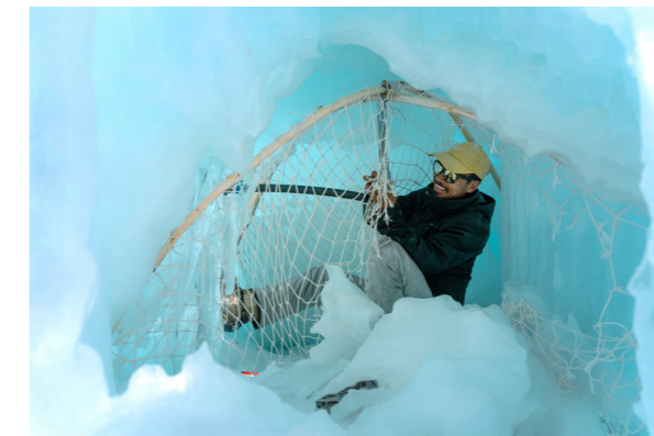
A fountain system sprays and freezes water in a domed structure
