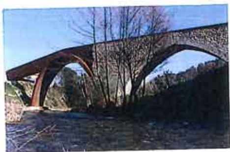
Bridge Xavier Font
