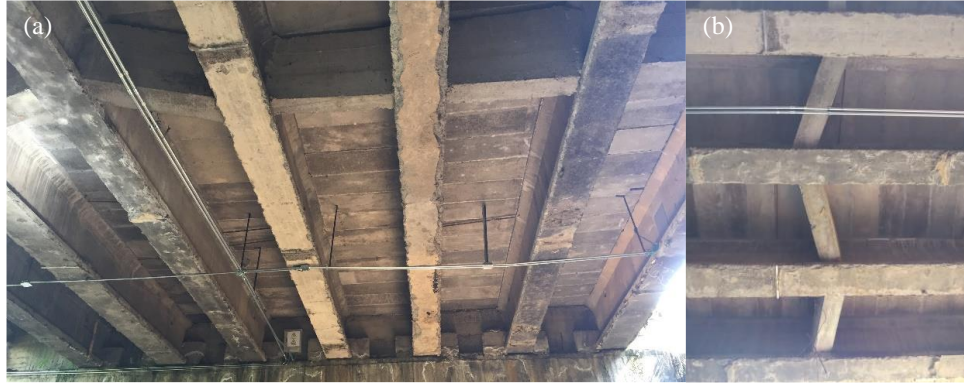
Fig. 14— Diaphragms at first third-span: (a) general view; (b) diaphragms between girders 1 and 4.
