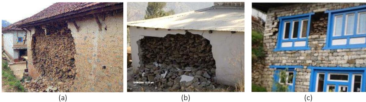
Figure 4.19: Delamination of external leaf of stone masonry wall due to out-of-plane effect (a) after 2015 Gorkha earthquake (Kuffel et al., 2015), (b) after 2005 Kashmir earthquake (Javed et al., 2006), (c) in Solukhumbu after 2015 Gorkha (Nepal) earthquake (Gautam et al., 2016)
