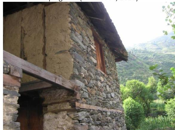
Figure 2.17: Wooden beam at lintel/floor level (Sood et al., 2013)
