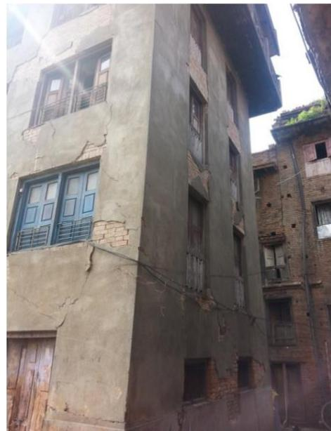
Figure 4.6: Spandrel failure (Shakya & Kawan, 2016)
