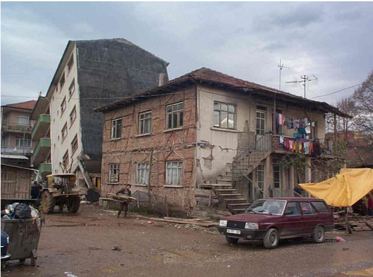
Figure 5.4: A *hımsı*, timber reinforced masonry house survived with very little damage next to a collapsed four-story RC building after the 1999 Duzce earthquake (Doğangün et al., 2006)
