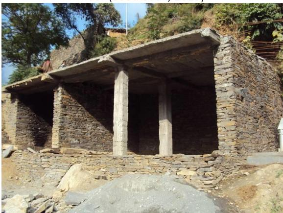
Figure 2.16: RC columns with stone masonry walls and RC slab floor (Sood et al., 2013)
