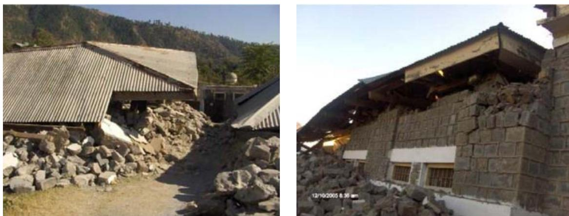
Figure 4.21: Failure due to lateral thrust from inclined roof (Naseer et al., 2010)
