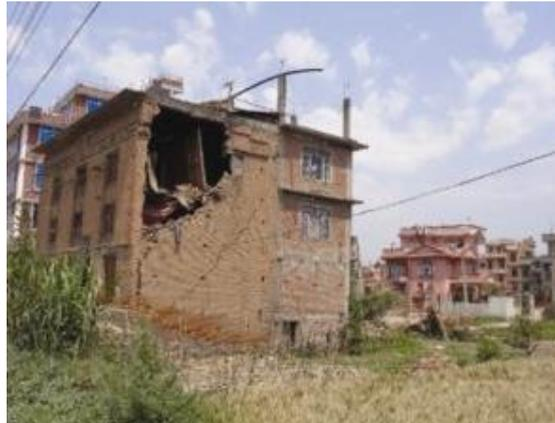
Figure 4.17: Combined in-plane and out-of-plane failure observed at Nikosera in unreinforced masonry after 2015 Gorkha earthquake (Rai et al., 2015)
