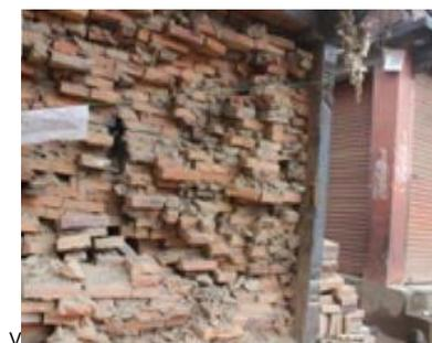
Figure 4.20: Masonry delamination due to (a)-(c) - absence of through stones. (d) - segregated mud mortar
