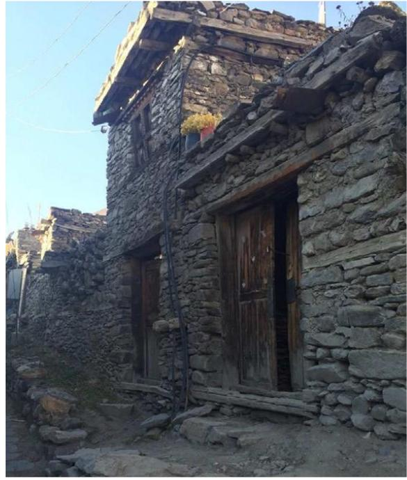
Figure 2.2: Typical Bhatar wall with dressed stone masonry (photo credit: Tom Whitty)
