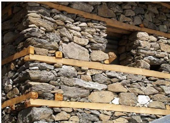
Figure 2.3: Taq wall with dry stone masonry (photo credit: Tom Schacher)
