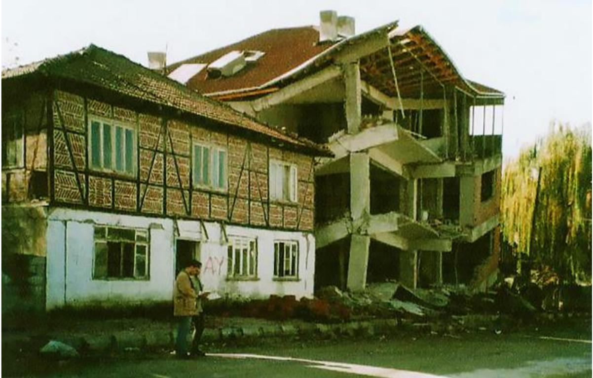
Figure 5.3: A *hımsı* building suffered relatively lesser damage whereas a 4 storeyed RCC building next to it suffered devastation with ground floor collapsing completely after the 1999 Duzce earthquake (Doğangün et al., 2006)
