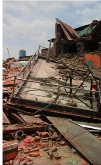
Figure 4.13: Collapse of RC slab on top of masonry walls (Gautam & Chaulagain, 2016)
