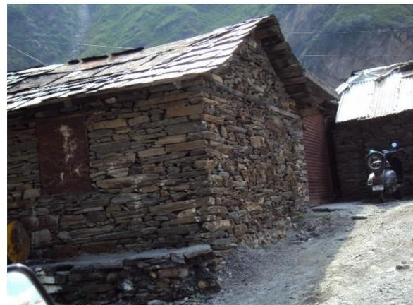
Figure 2.15: Dry stone masonry wall with stone slate sloping roof (Sood et al., 2013)
