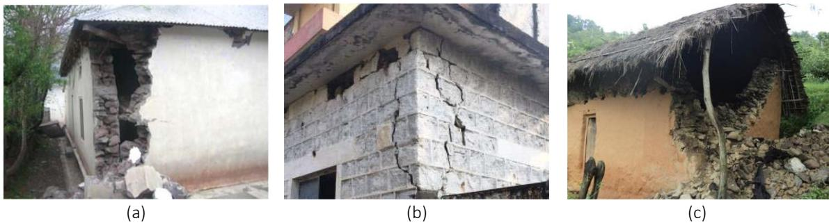
Figure 4.18: Corner damage (a) in Muzaffarabad after 2005 Kashmir earthquake (Naseer et al., 2010), (b) in unreinforced stone masonry building after 2015 Hindukush earthquake (Ismail & Khattak, 2016) (c) in stone masonry building after 2011 Sikkim earthquake (Gautam et al., 2021)
