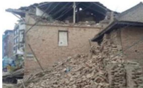
Figure 4.11: Out of plane collapse and overturning of gable masonry (a) (Javed et al., 2006) (b) (Gautam et al., 2016)
