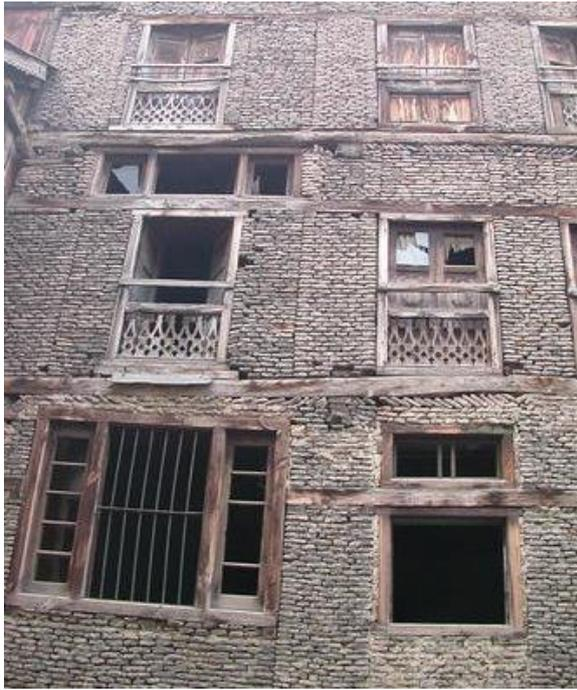
Figure 2.1: Taq building with horizontal timber bands and brick masonry (Jain, 2016)
