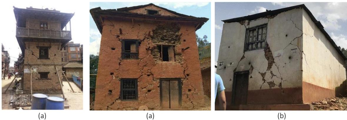
Figure 4.1: In-plane shear damage in walls with openings in (a) in brick masonry building (Shakya & Kawan, 2016), (b) and (c) Stone masonry buildings (Adhikari & D'Ayala, 2020)
