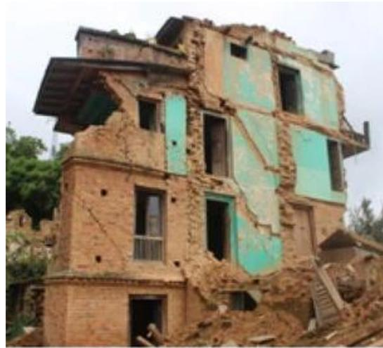
Figure 4.10: Out-of-plane collapse of majority of walls (Gautam et al., 2016)
