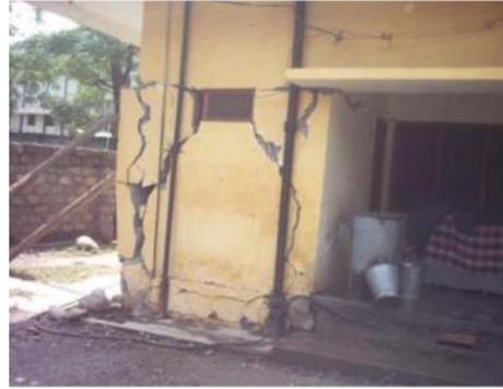
Figure 4.16: Combined in-plane and out-of-plane failure observed in Kashmir after 2005 earthquake (Naseer et al., 2010)
