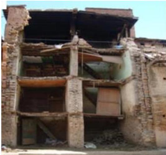
Figure 4.9: Complete collapse of façade (Gautam et al., 2016)
