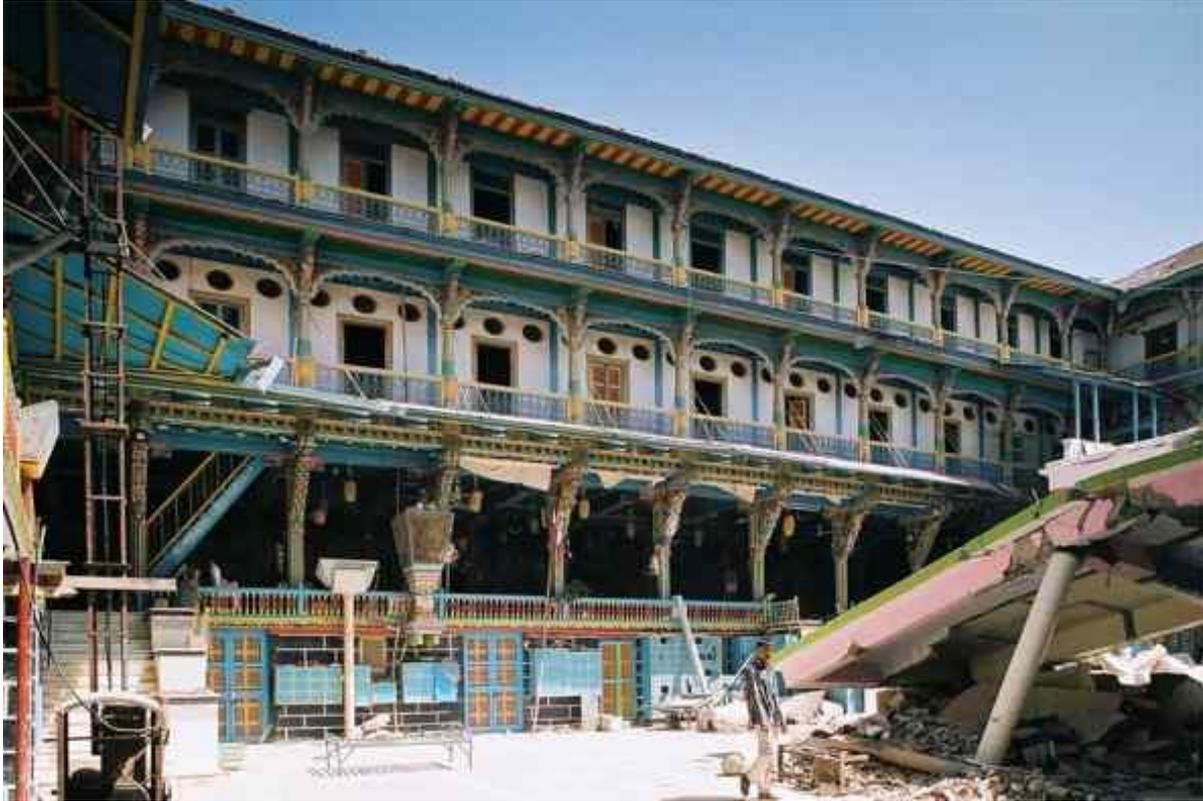
Figure 5.5: Only minor hairline cracks were noticed in the 150 year old timber-masonry Swaminarayan Temple while more modern RCC structure in the complex (visible in the front) collapsed completely after the 2001 Bhuj earthquake (Photo credit : Randolph Langenbach)
