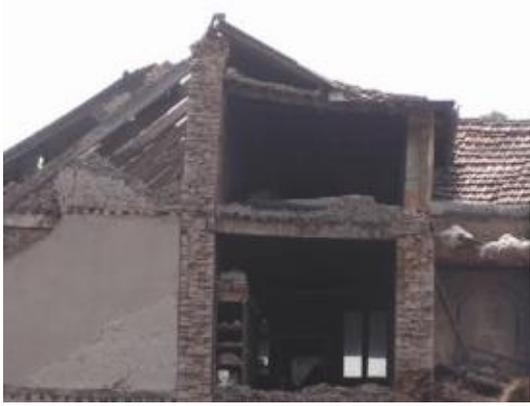
Figure 4.12: OOP collapse of wall due to inadequate connection with roof floor and transversal wall (Rai et al., 2015)
