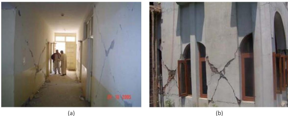
Figure 4.2: (a)-(b) - Diagonal shear failures of masonry wall piers (Naseer et al., 2010)
