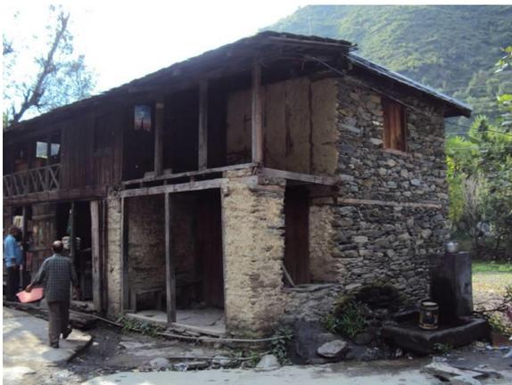
Figure 2.14: Dry stone masonry walls with wooden floor (Sood et al., 2013)
