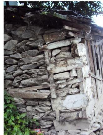
Figure 2.11: Thola with stone masonry infill within (Rahul et al., 2013)
