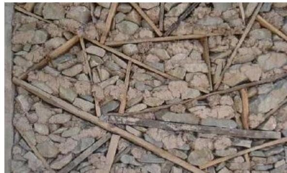
Figure 2.8: Random patterns in timber bracing, possibly to use available sizes of wood (Hicyilmaz et al., 2009)
