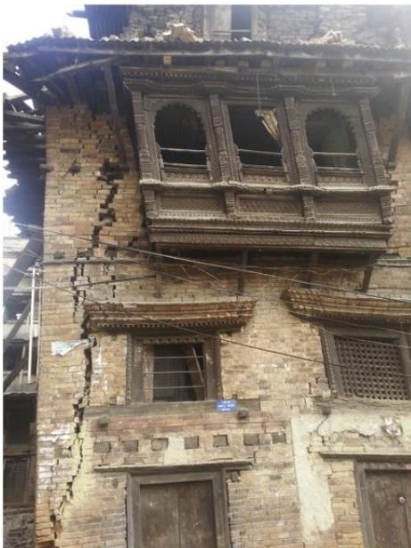
Figure 4.5: Tension failure of building (Shakya & Kawan, 2016)
