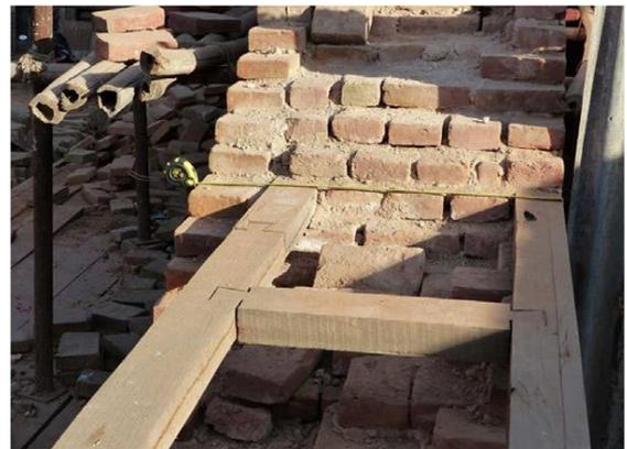
Figure 2.4: Timber ladder (band) with brick masonry (photo credit: Martijn Schildkamp)
