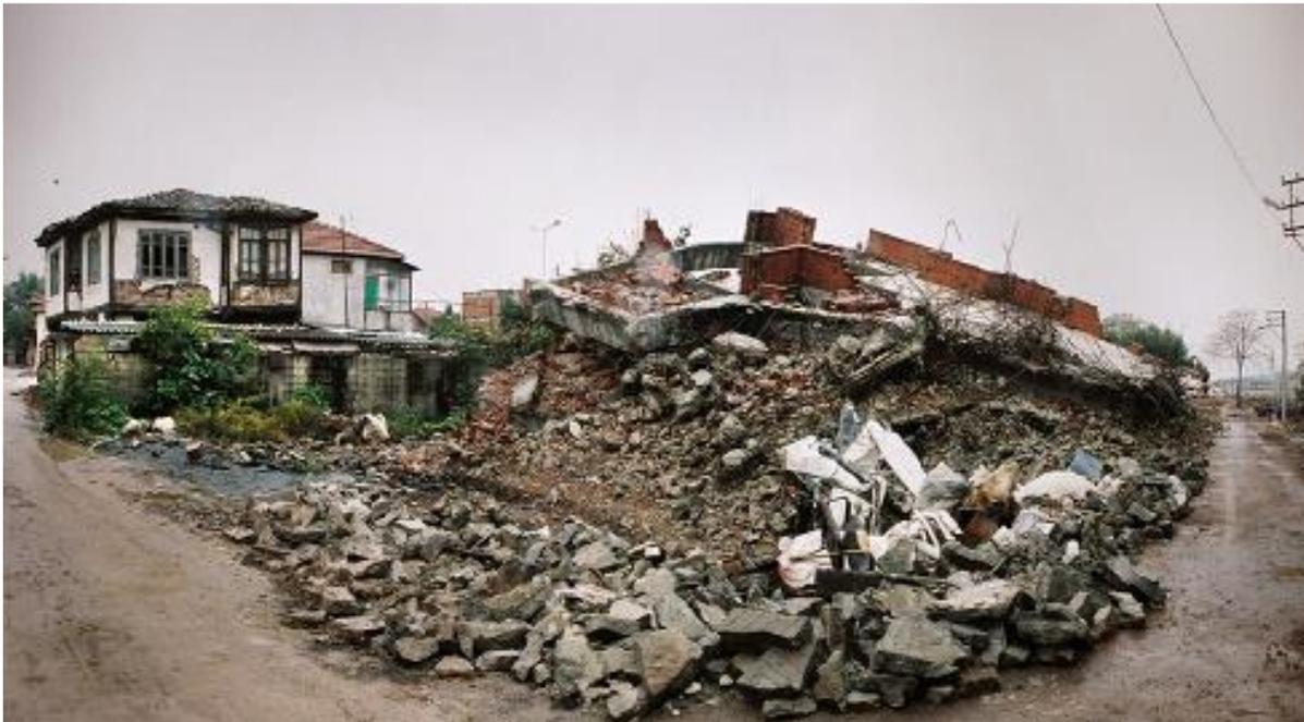
Figure 5.2: A traditional timber-reinforced *himiş* building standing in the backdrop while several multi-storeyed modern RCC buildings suffered pancake collapse in Adapazari after the 1999 earthquake (Langenbach, 1999)
