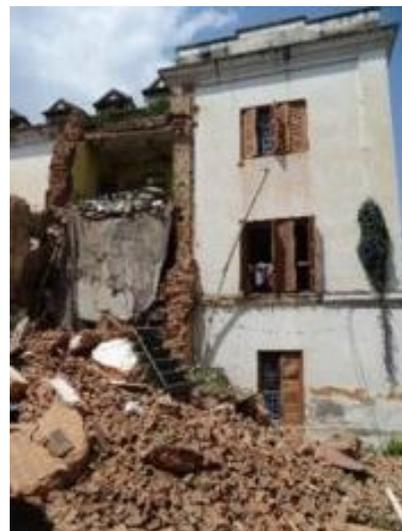
Figure 4.15: Out of plane damage due to asymmetrical plan or protruded part of the building (Dizhur et al., 2016)
