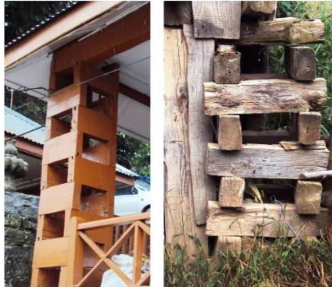
Figure 2.9: Thola columns in Thathara house(a) Thola in a modern construction. (b) An older thola column with rudimentary, unfinished planks and unsophisticated joinery (Rahul et al., 2013)
