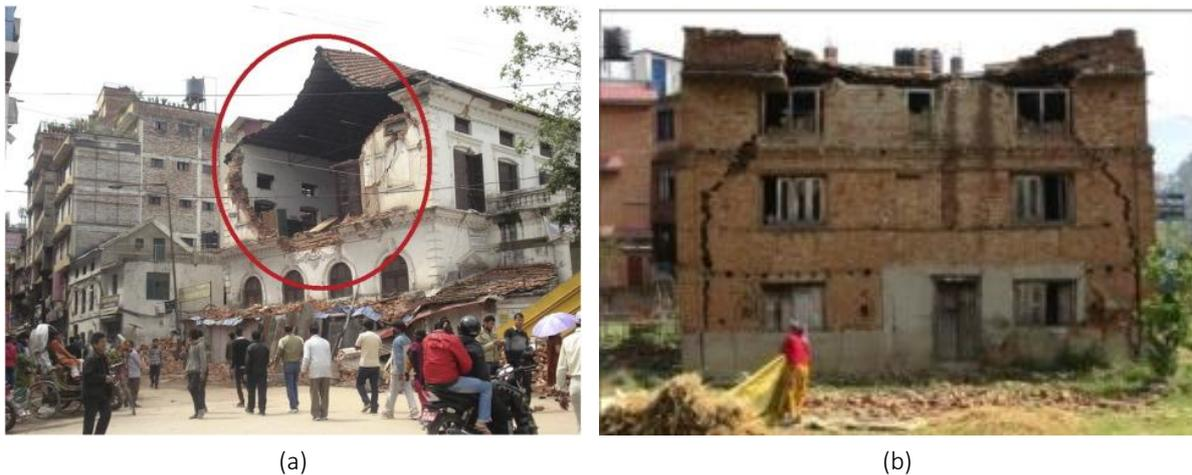
Figure 4.7: (a) – (b) Out of plane collapse of façade wall (Dizhur et al., 2016)
