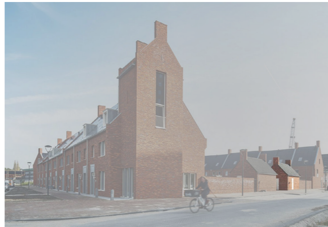
Image 6.4: Example of transformer house in the same design as the surrounded houses
