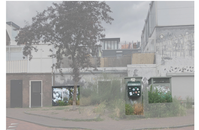
Image 6.5: Different transformer houses close to each other.
