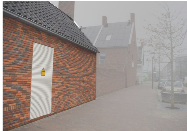
Image 6.3: Example of transformer house in the same design as the surrounded houses
