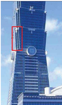
Figure 3-52 Taipei 101 corner modification
