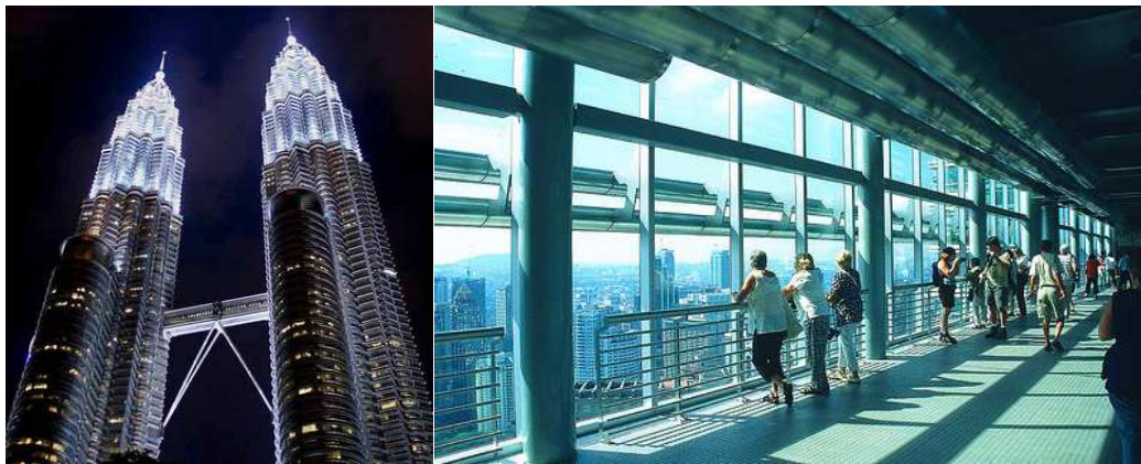
Figure 3-29 Petronas Towers and skybridge (no structural link)
