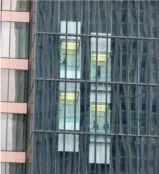
Figure 3-56 double decker lift Midland square, Nagoya
