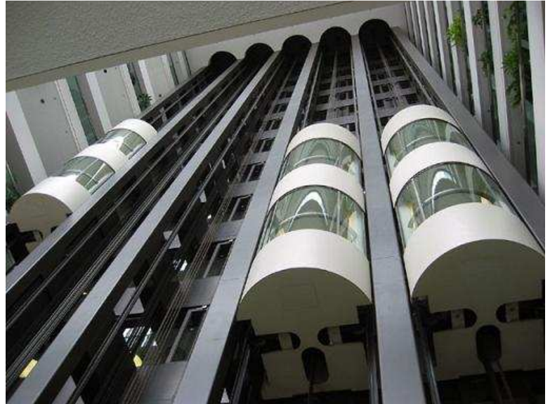
Figure 3-57 double decker lift- Midland square,Nagoya
