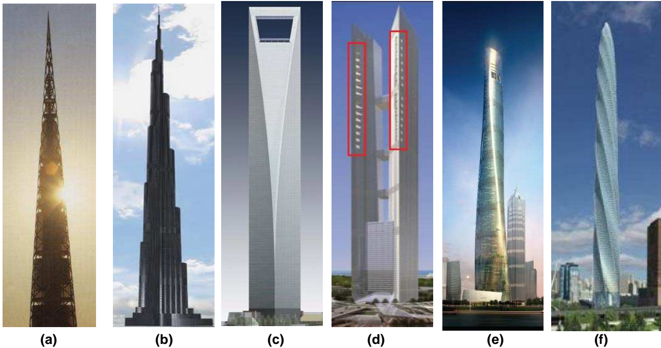
Figure 3-53 Examples of wind-reducing building shapes
