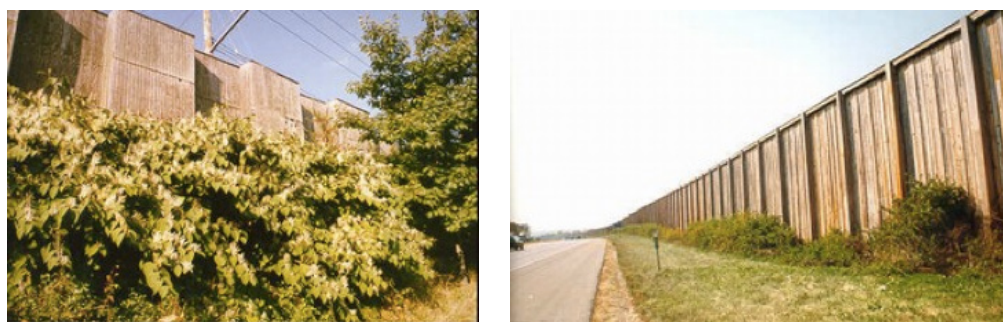
Figure C3.5: Ply and GL wood barriers.
