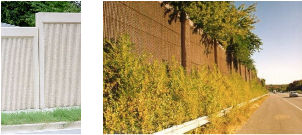
Figure C3.1: Concrete noise walls.
