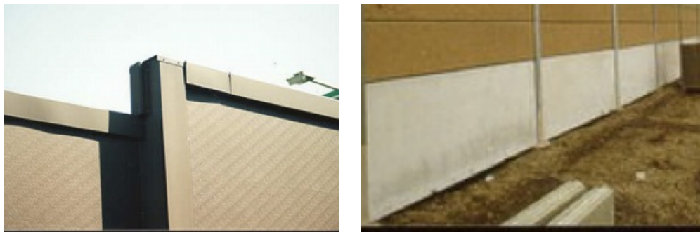
Figure C3.8: Plywood with fibreglass skin barriers.
