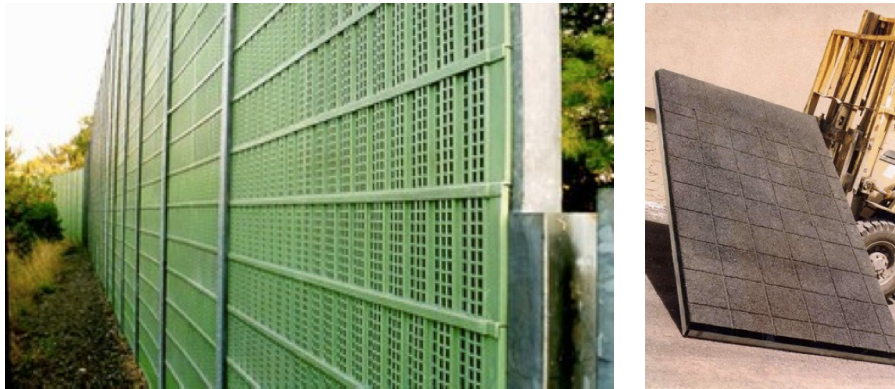
Figure C3.7: Fibreglass (left) and recycled plastic (right) barriers.
