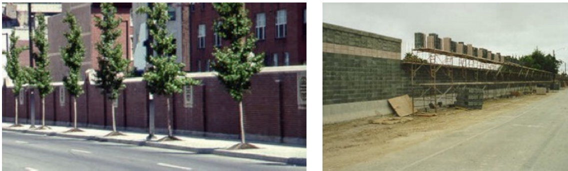
Figure C3.2: Brick and masonry block barriers.
