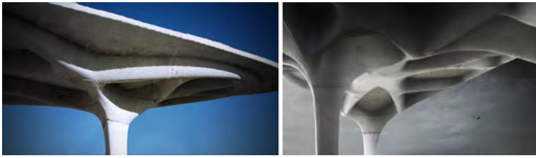
Figure 3.22: Topology-optimized concrete prototype from the Unikabeton project, produced via robotic CNC milling of EPS molds
