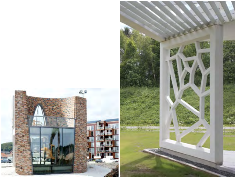
Figure 4.10: Left Recently completed mock-up of the Kirk Kapital HQ, for which the formwork was realized by robotic means by Odico formwork robotics Right Architectural elements produced by robotic means, deriving toolpaths from STEP data
