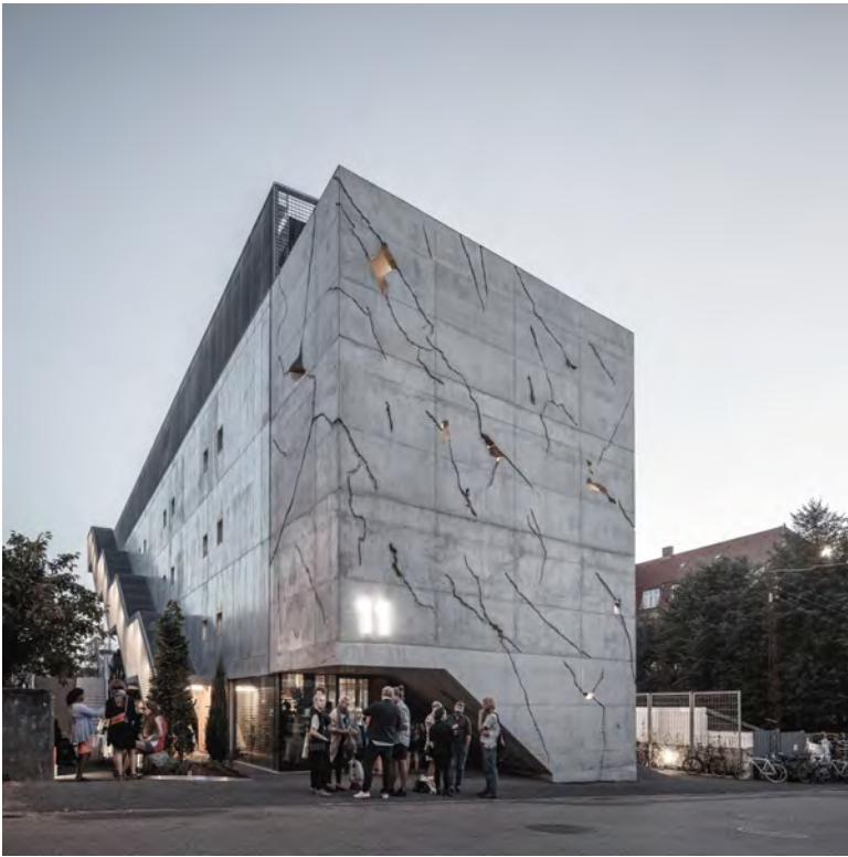
Figure 4.1: Robotic hot-wire-cut façade patterns and apertures for the in-situ cast concrete façade of the Sonnesgade 11 mixed use complex, Aarhus, by Sleth Architects Photo: Rasmus Hjortshøj
