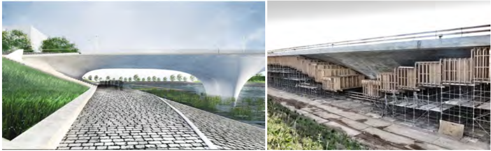
Figure 3.7: The Waal Bridge Extension Impression of the artist (left) (©Zwart & Jansma) Construction work using traditional formwork systems (right)
