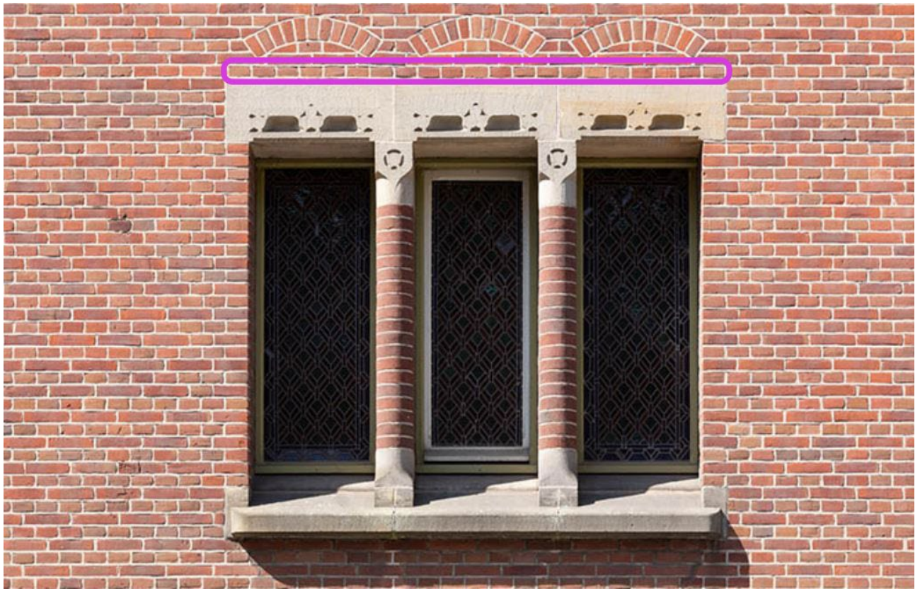
Figure 10 – 21 brick heads above a window opening in the Beurs façade, edit from author (van Hoek, Bart n.d.)
