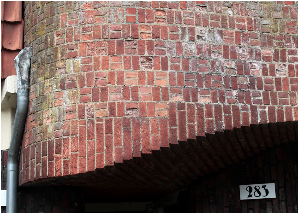
Figure 2 - Detail of brick overhang in Het Schip (Hidden Architecture 2015)
