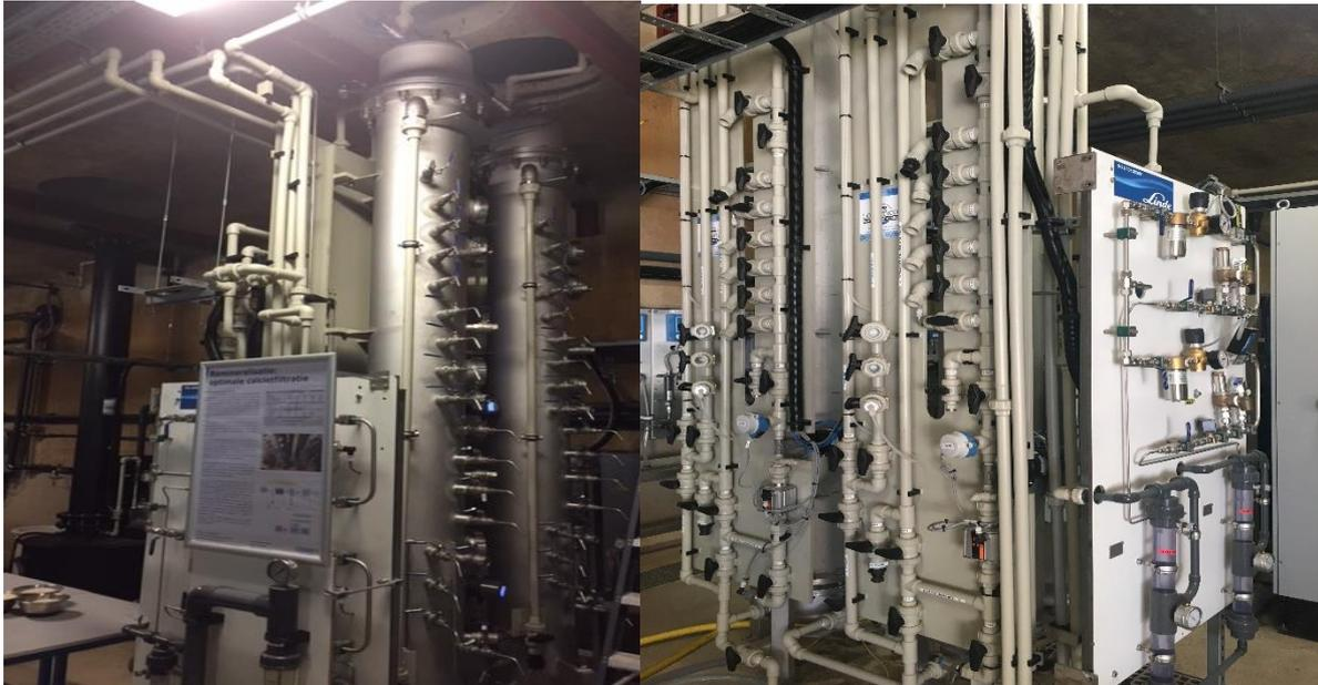
Figure 6. Photo of pilot calcite filter at Kamerik, both from the front and the back
