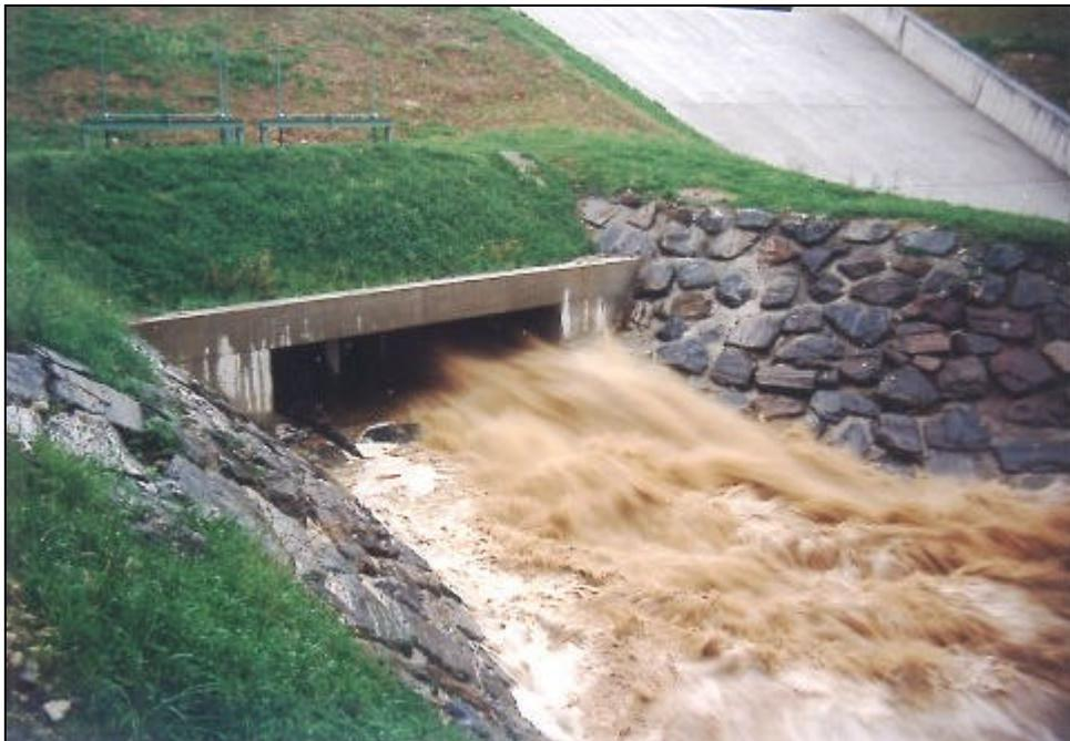
**Figure 3.3.2.2 h** – Bottom outlet of retention basin in Styria
