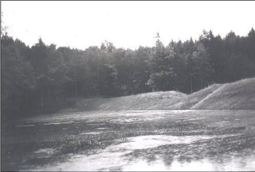
**Figure 3.3.2.2 e** – Retention basin in Styria during a flood event
