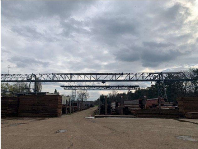
Where elements are unloaded:
