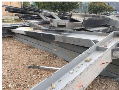
Figure 15: damaged beams (Terwel et al., 2021b)
