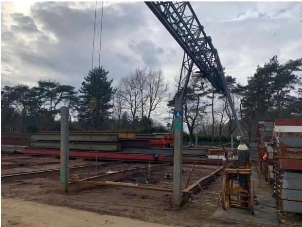
Storage of beams:
