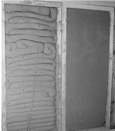
2.6.21, 22 structural elements filled with loam German firm HDB Weissinger produces 1m wide and up to 3 m high timberframe wall elements filled with lightweight loam ( Minke, 2006 )
