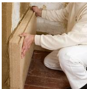
2.6.24, 25, 26 Prefabricated panels of loam ( baksteen.be/nl.html )
