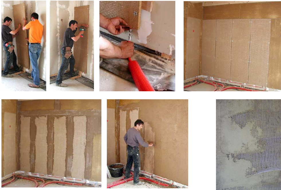
3.2.31,32,33,34,35,36 steps of installation and finishing surface ( wall-heating.com )
