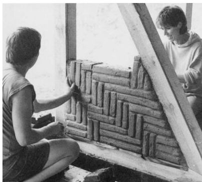
2.6.23 using earth with timber frame structure ( Minke, 2006 )
