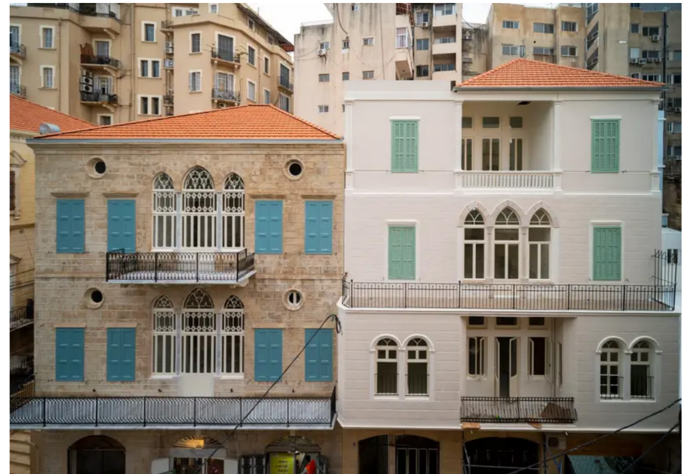
Figure 25 Refurbishing damaged heritage buildings (Issa, 2022)
