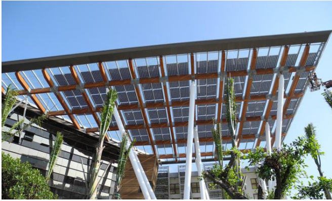
Figure: I64. Lamboo used outdoor in solar roof
