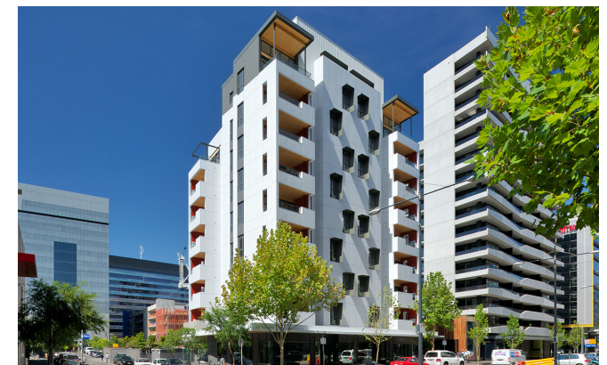
Figure:48. Forté Building
