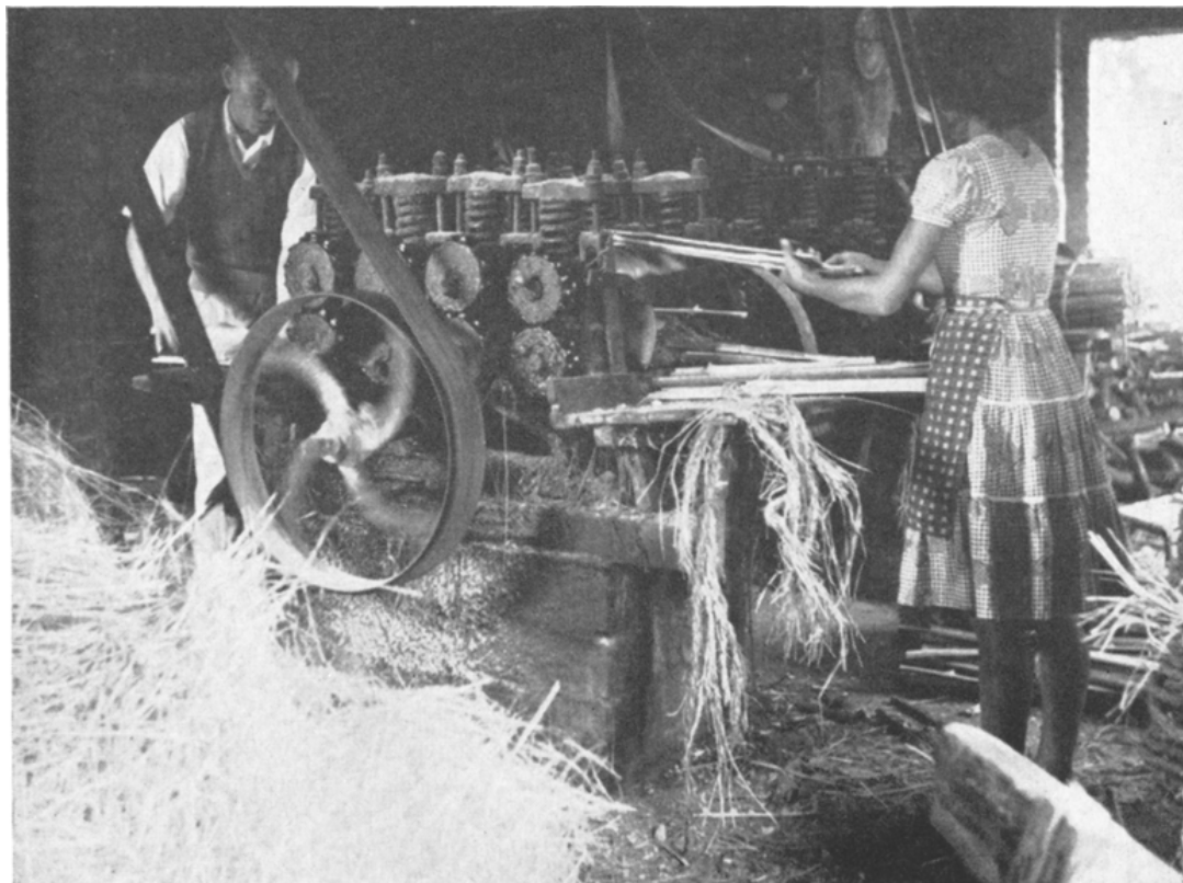
Figure:60. Machine making bamboo fibers
