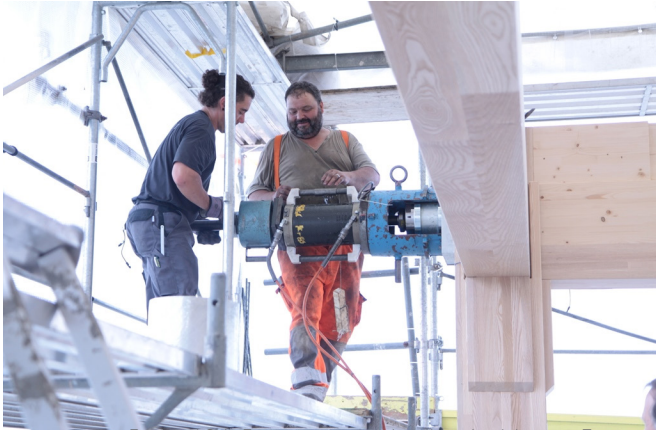
Figure: 124. First prestressed timber building in Europe (near completion)
