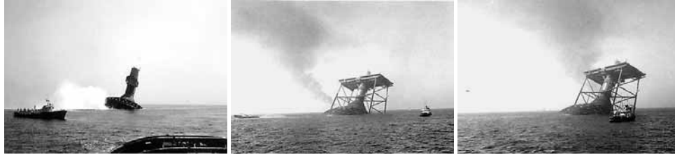
Figure 1.9: Installation of Khazzan Dubai storage tank No. 1
