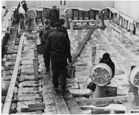
Figure 1.3: Construction of the scale model of the Habbakuk in ice (left) and the final full-scale design compared to an aircraft carrier and battle ship (right)
