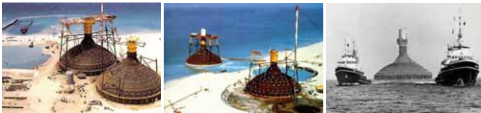
Figure 1.7: Construction and towing of the Khazzan Dubai storage tanks
