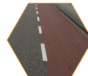
Asphalt and cycling lane
