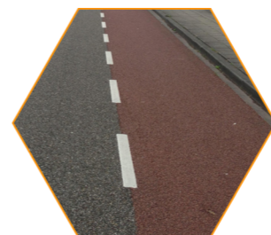
Asphalt and cycling lane
