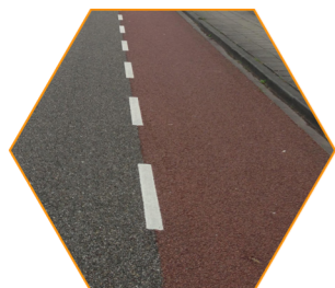
Asphalt and cycling lane
