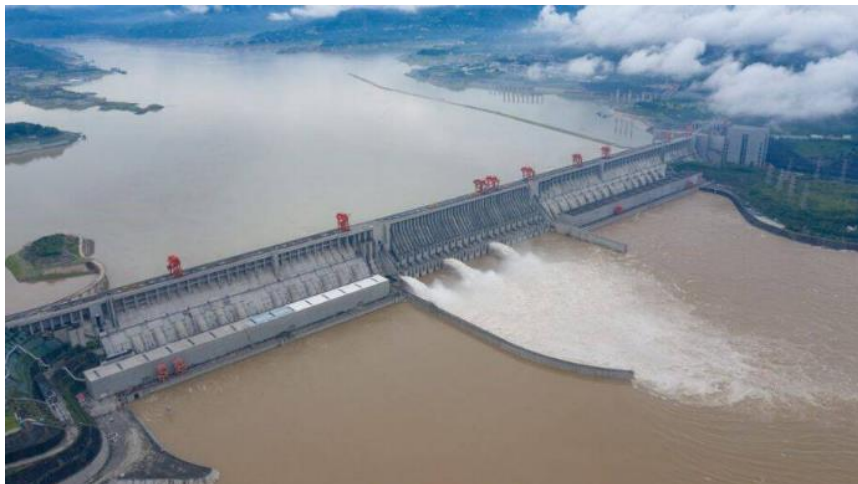
Figure A - 2 Three Gorges Dam, China. This is an open-loop storage, because there is a natural flow into the upper reservoir from the Yangtze River (Asia News, 2020).
