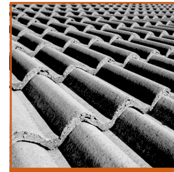
Roof tiles, teglageret 220 km
