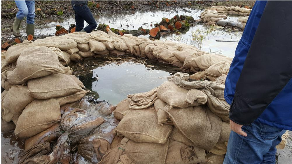
**Figure 3-4:** Ring dam around a sand boil at the river Waal, Netherlands. A ring dam serves the purpose to decrease the head across the dike and thereby stop further erosion. Source: J.C. Pol
