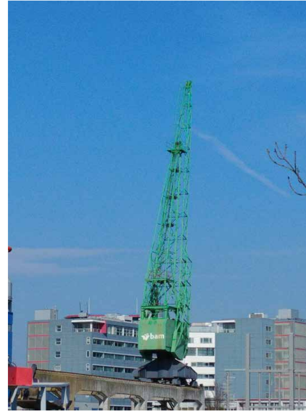
Images | Cranes at the HAC terrain
