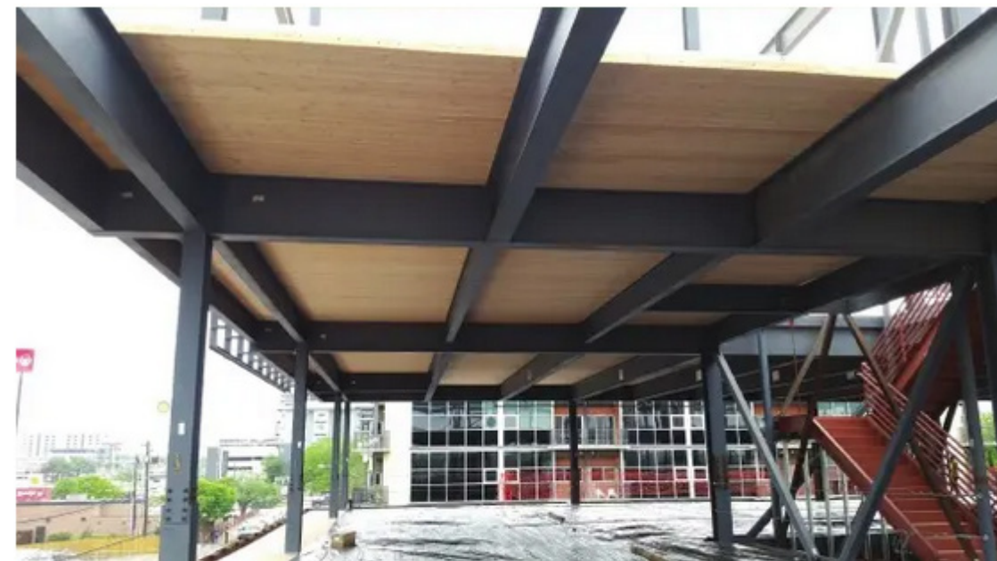
Fig. 2-8. CLT panels supported on steel beams (photo courtesy of David Barber).
