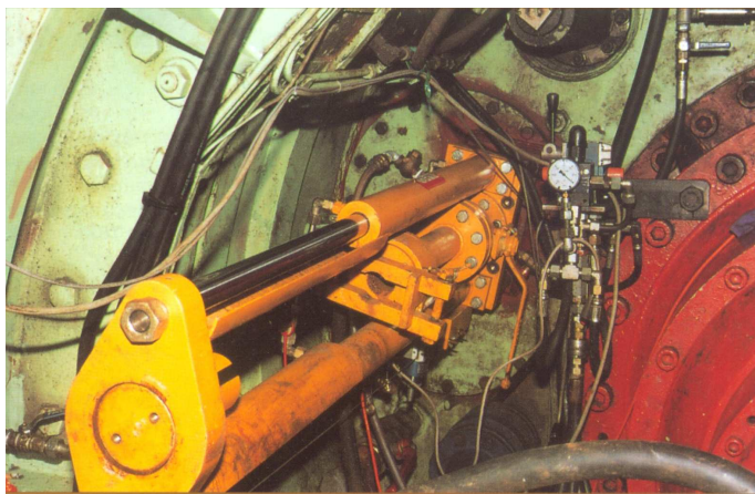
Figure 2. HCPT rig installed in a pipe jacking TBM.
