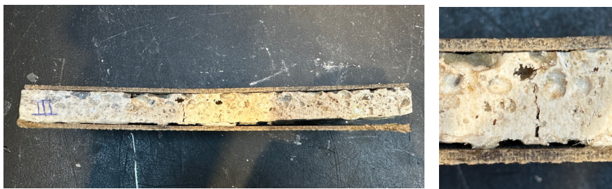
Figure 107: Images of PLAX B2. Left; Image after the testing testing; Right, close up where the material has failed.
