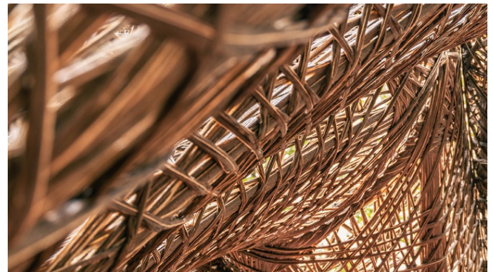
Figure 17: Natural fibers construction. (Natural Fibre Structures, Cluster of Excellence Integrative Computational Design and Construction for Architecture, University of Stuttgart.
