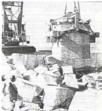
Figure 4-18 Block clamp for the breakwater of Scheveningen
