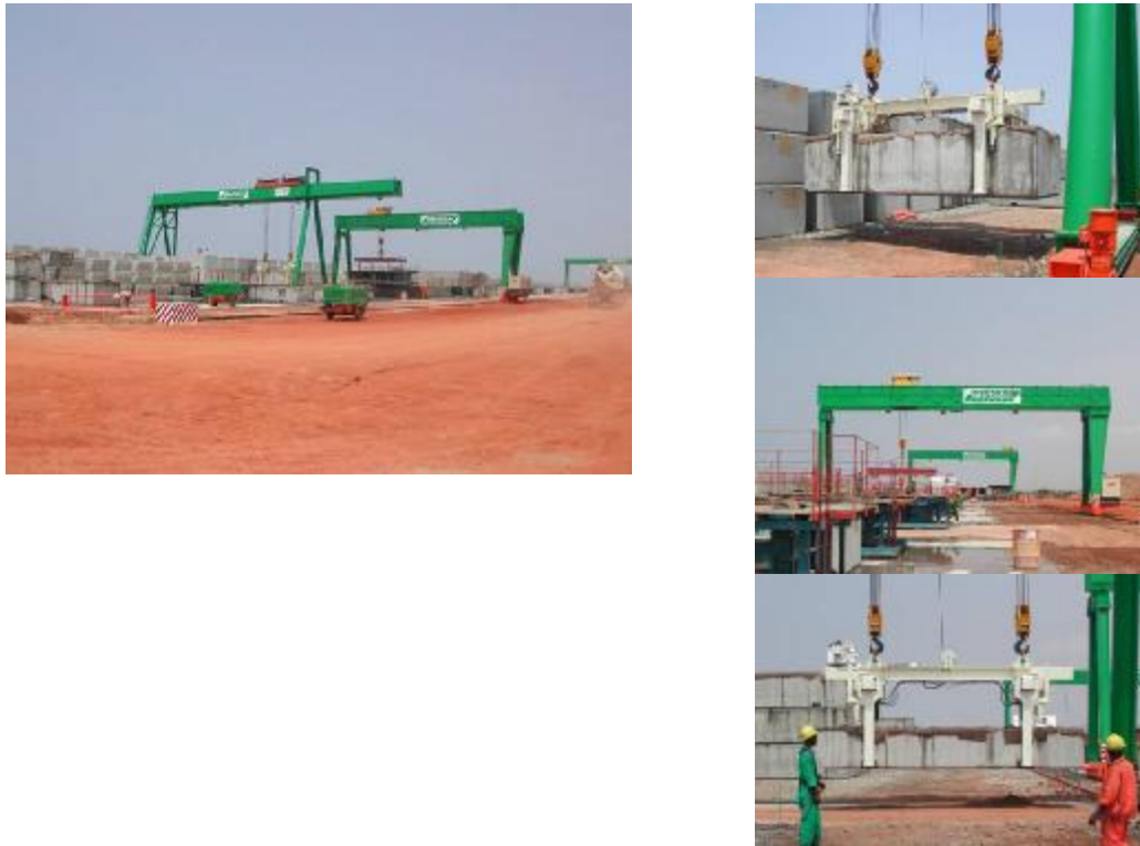
Figure 5-9 Lifting of concrete units
