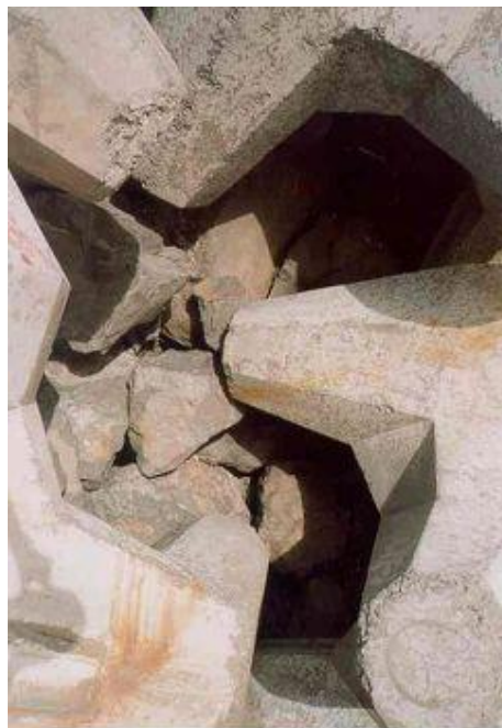
Figure 8-14 Gap in berm
