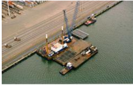
Figure 2-18 Crawler crane on pontoon; Photograph Stemat
