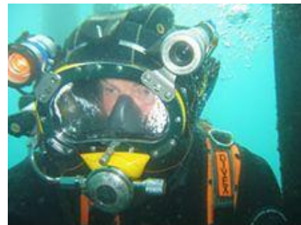
Figure 2-26 Inspection by diver with light and camera
