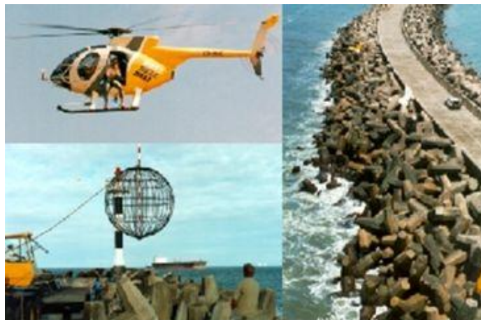
Figure 2-28 Digital imaging by helicopter; Crane and ball survey, photograph CSIR
