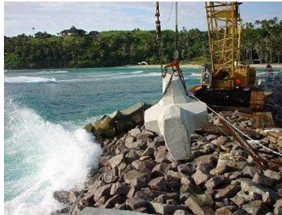
Figure 2-13 Placing of Accropodes with sling on Fregate Island; Photograph DMC
