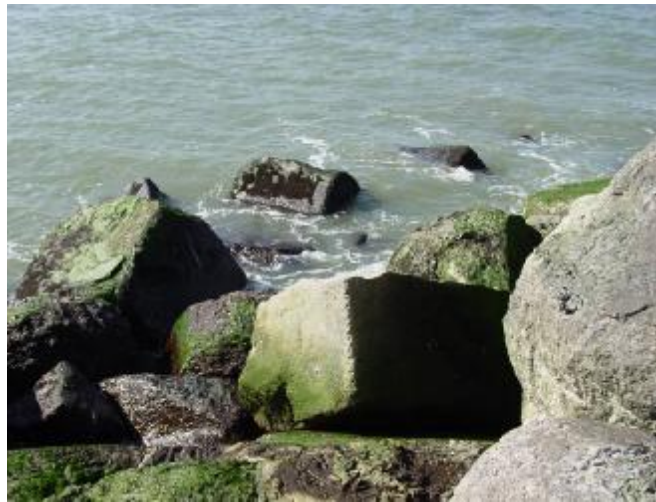
Figure 3-4 Poor concrete quality of the cubes
