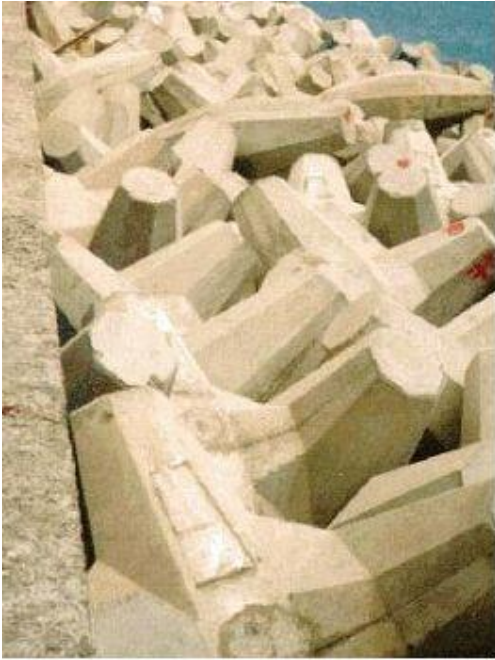
Figure 8-12 Correct placement
