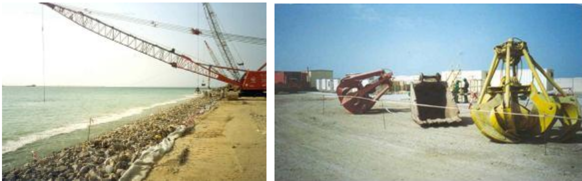
Figure 2-12 Left: Crane topping of to reach outside berm Right: Orange peel grab
