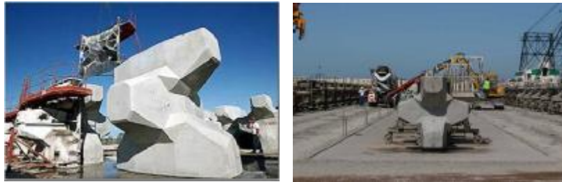
Figure 5-5 Casting of Accropodes
