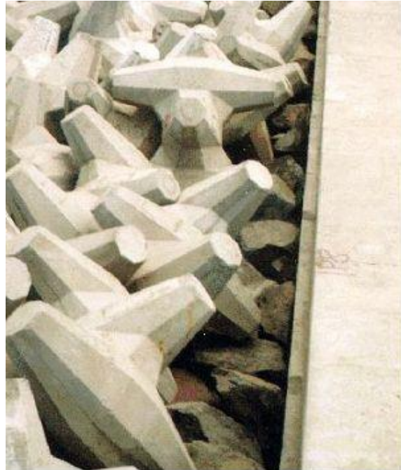
Figure 8-13 Gap with crest wall
