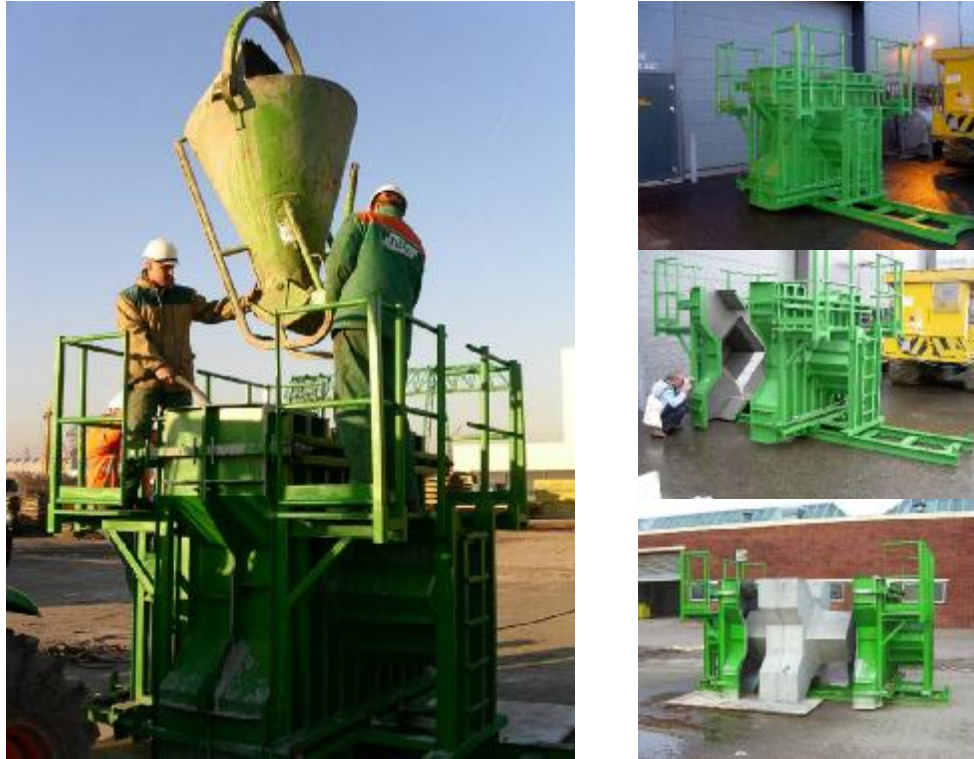
Figure 5-7 Casting of Xblocs
