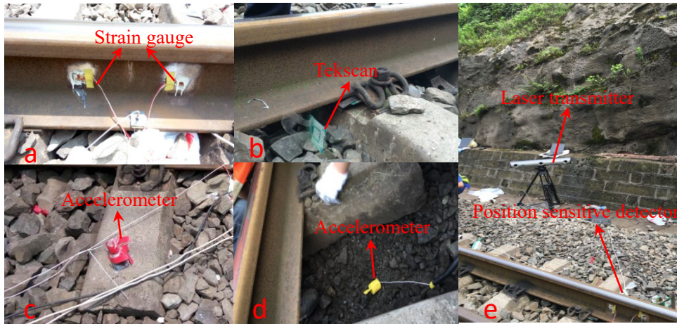
Fig. 6 Detail of track instrumentation at transition zone: (a) dynamic load on rail; (b) rail seat loads; (c) sleeper acceleration; (d) special box for accelerometer in ballast bed; (e) sleeper displacement
