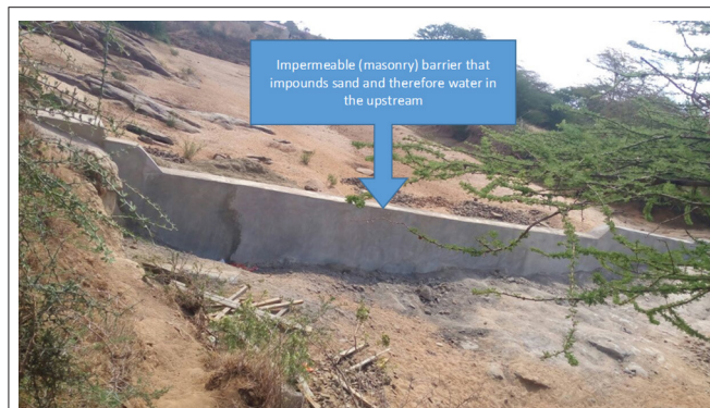
FIGURE 4 | A newly built sand-storage dam.
