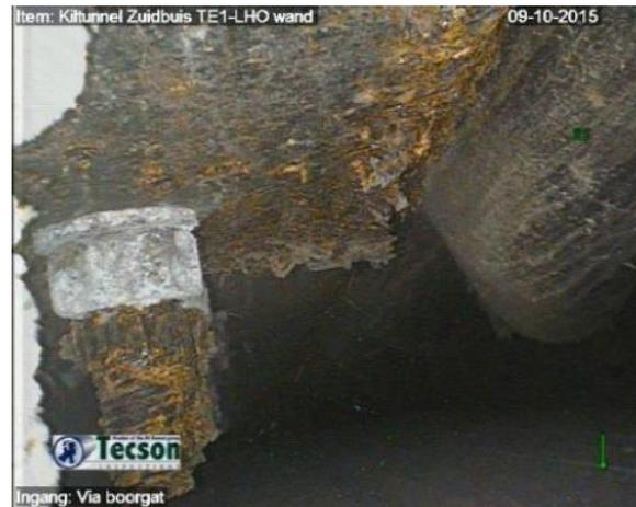
Figure 43: Corroded clamping structure at the wall of the Kil Tunnel, from the research in 2015 (Leeuw, 2015)
