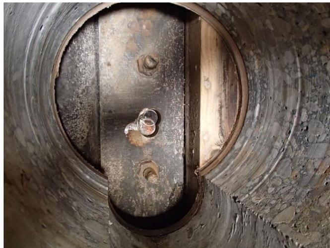
Figure 25: Picture of the clamping structure of the Omega-seal in the Kil Tunnel, which can only be seen by making a large hole in the concrete fill (COB, 2017)
