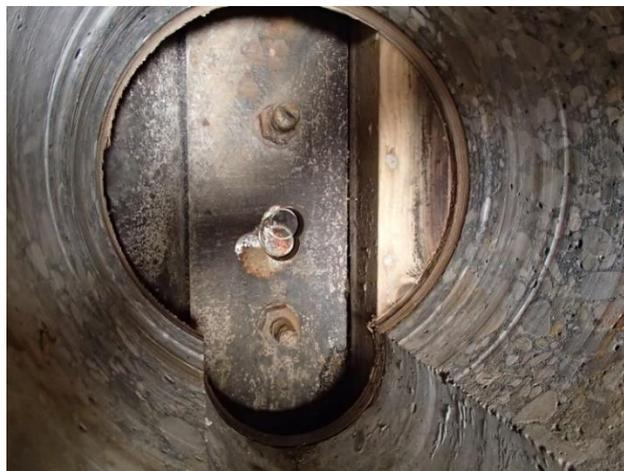
*Figure 45: Clamping plate, with stud through it, seen from the tunnel tube (COB, 2017)*
