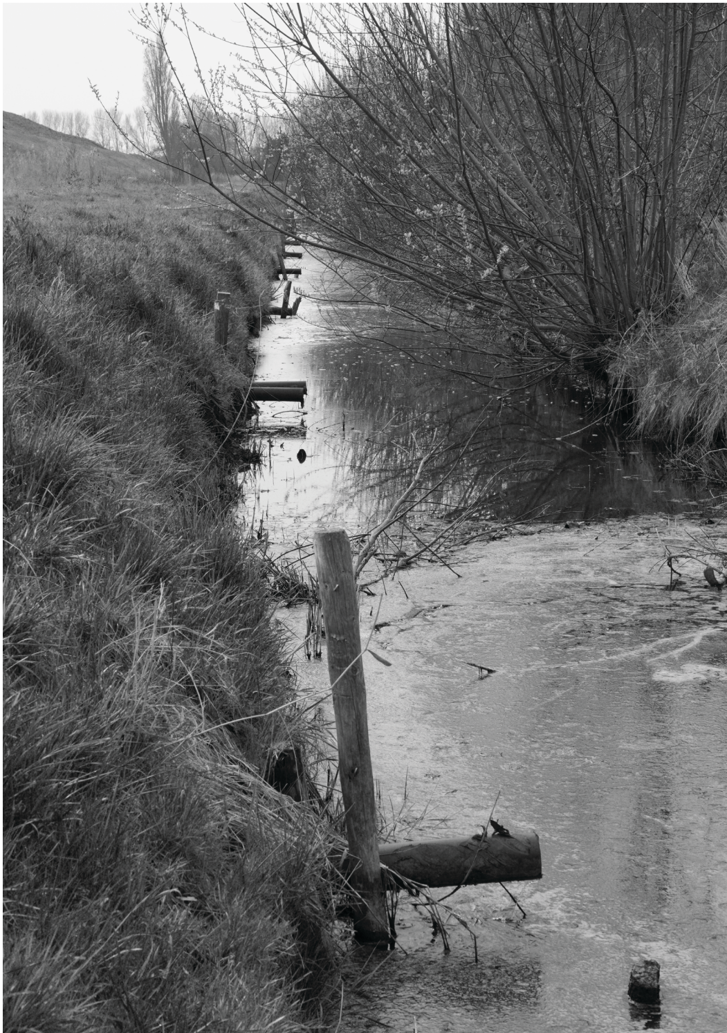
Fig. 1 Drainage outlet from the ash mound to the adjacent drainage canal, showing the existing water management system (Source: Pelin Yalçın, 2026).
