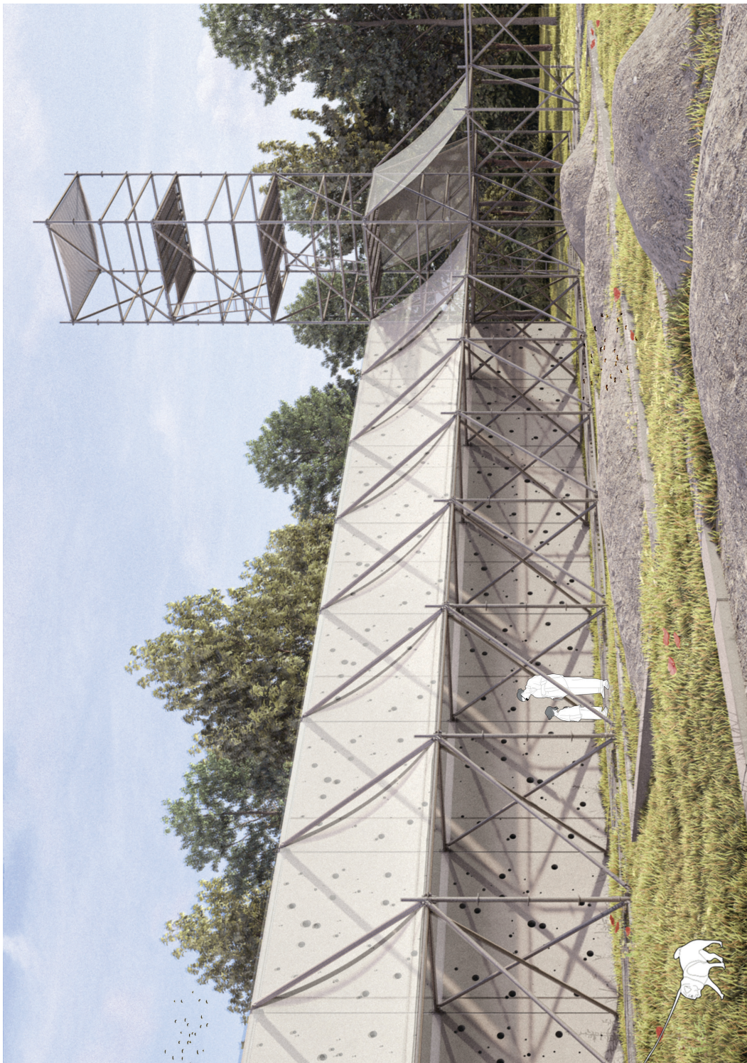
Fig. 44 View of the Bee Pavilion, showing perforated ash-concrete blocks and a scaffolding observation tower placed within the landscape. The pavilion works as both habitat and public learning structure, allowing pollinators to inhabit the wall while visitors observe the ecological role of the parcel (Source: Pelin Yalçın, 2026).
